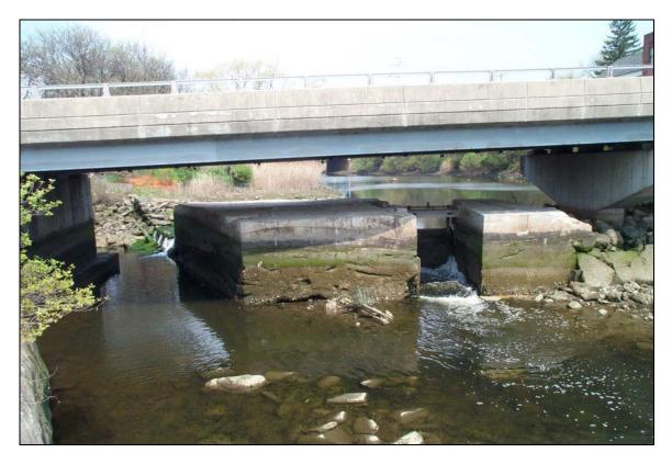
Plate 8. Concrete obstruction under Pulaski Street Bridge on the Mill River in Stamford, CT. This abandoned structure blocks fish passage during mid and low tides.
