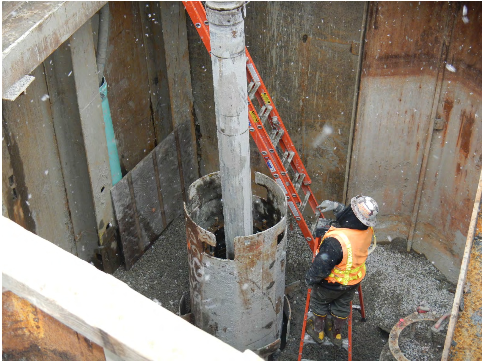
Concrete placement of drilled shaft at the downstream northeast wing wall of the new Brookline Avenue Culvert – early March 2016.
