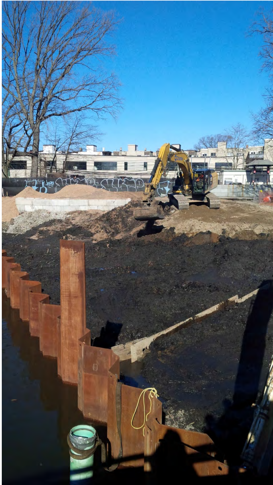
Excavator mixing saw dust into the river sediment to help solidify the material for transport off-site – upstream of the existing Riverway Intake Structure – mid February 2016.
