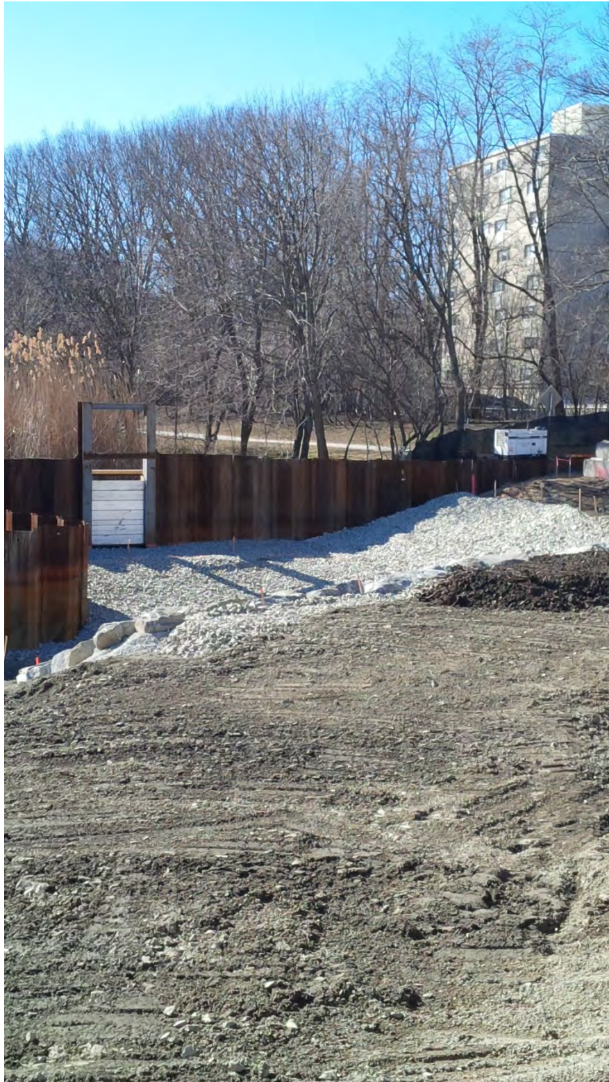
Constructed FRM channel downstream of the Flow Restriction Control Structure (FRCS) at the Riverway – note the stone protection on the excavated bottom and bank of the channel – early March 2016.
