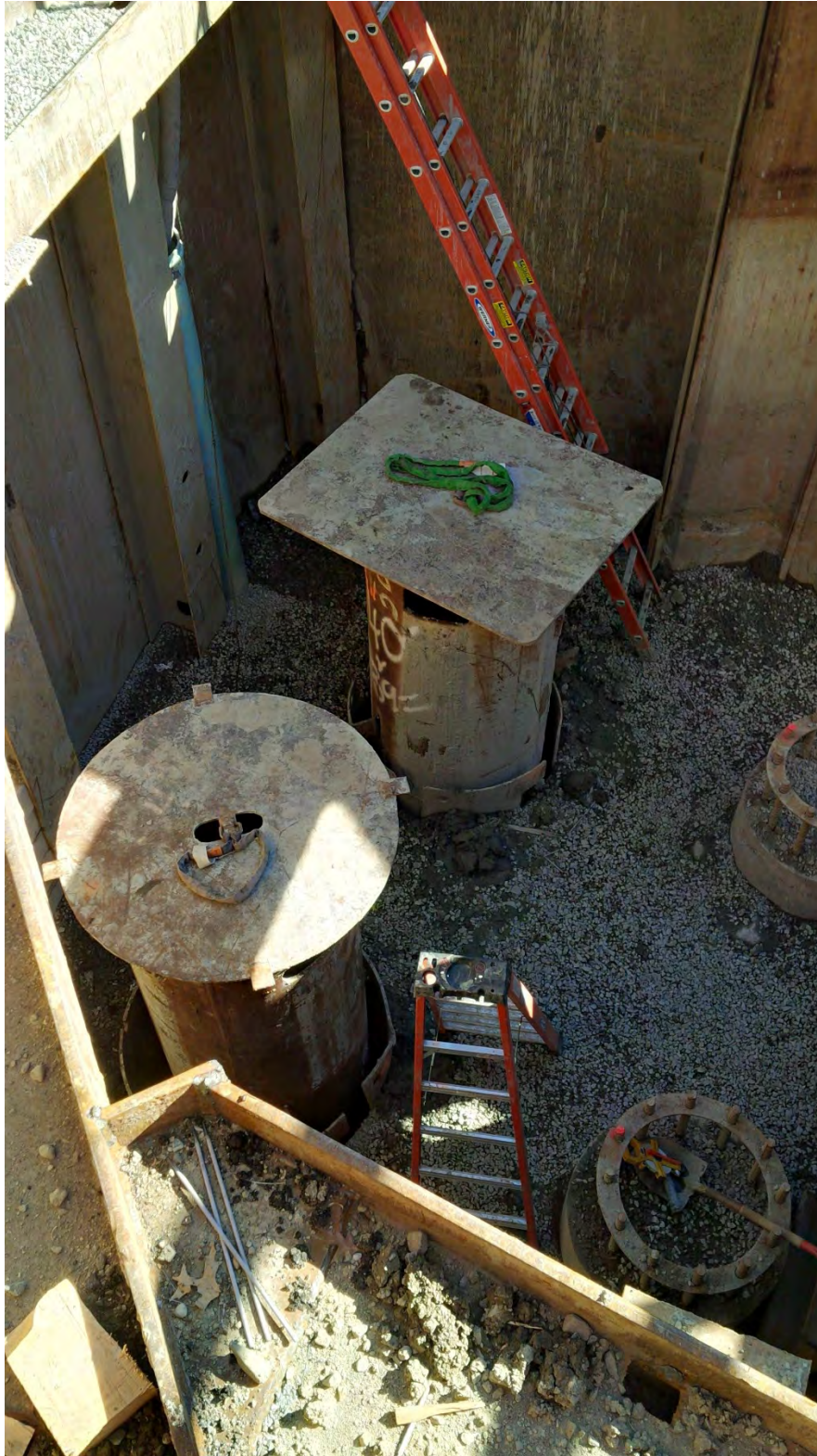
Last remaining two drilled shafts at the downstream northeast wing wall of the new Brookline Avenue Culvert – the hole has been drilled to depth and awaiting concrete – early March 2016.
