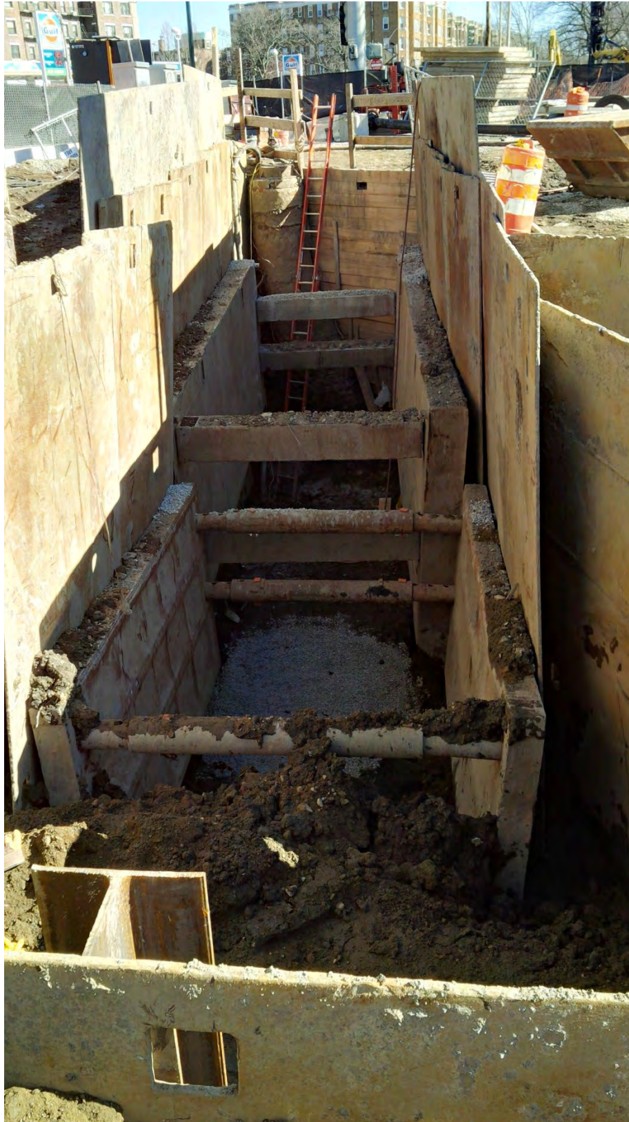
Area upstream of the new Brookline Avenue Culvert – excavation to install the new relocated sewer line. Note the existing manhole on the far side (adjacent to the ladder) that the new line will connect to – early March 2016.
