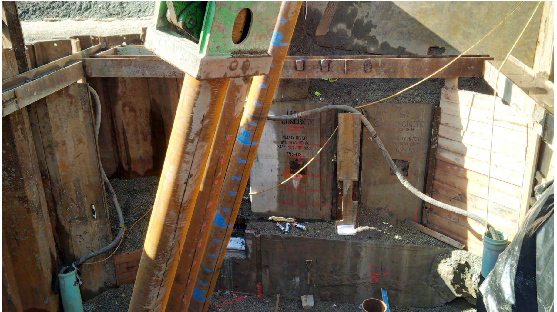
Downstream Riverway Culvert work area – area has been excavated to bottom of pile cap and the vertical steel pipe piles have been installed. Note the battered steel pipe piles are being installed – mid March 2016.
