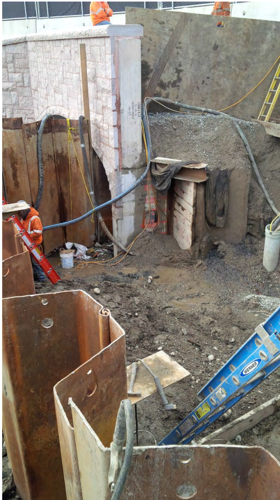
Support of Excavation (SOE) installed in order to excavate down to grade for the new northeast wing wall at the downstream of the new Riverway Culvert – early March 2016.
