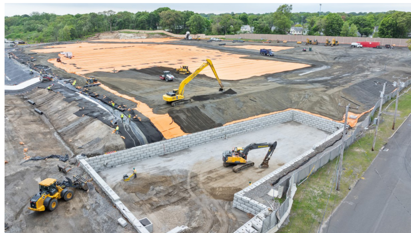
Raymark Superfund Site, Stratford, CT Hazardous waste cap at Operable Unit (OU) 4
