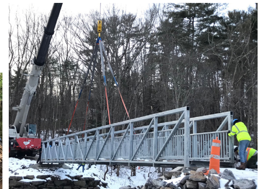
Installation of Bridge, West Thompson Lake, CT
