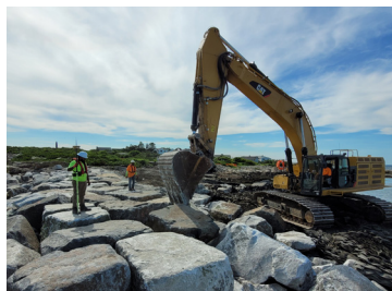
Breakwater Repairs, Isle of Shoals, NH & ME
