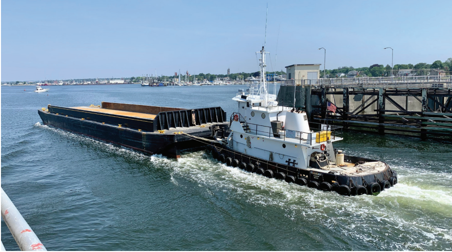
A vessel travels through the New Bedford Hurricane Barrier.
