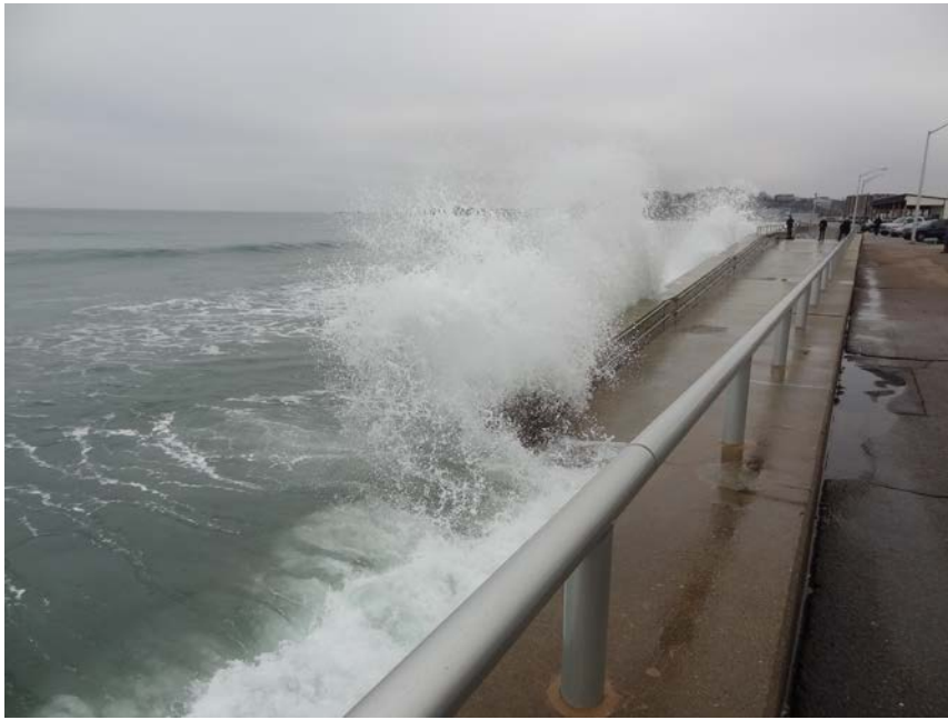
Photo 7 Waves overtop the sea wall in front of the DCR bath house.
