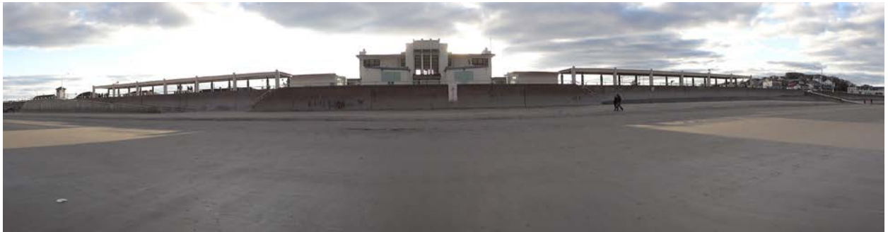
Photo 1 A view of the south end of the sea wall in Zone 2 with the DCR bath house and other public infrastructure behind it.
