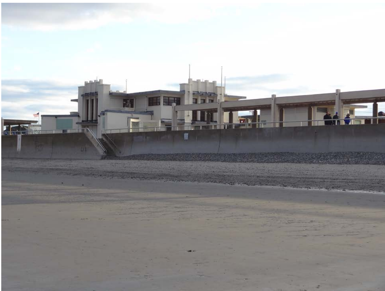
Photo 5 The DCR bath house is located very close to the sea wall in Zone 2.
