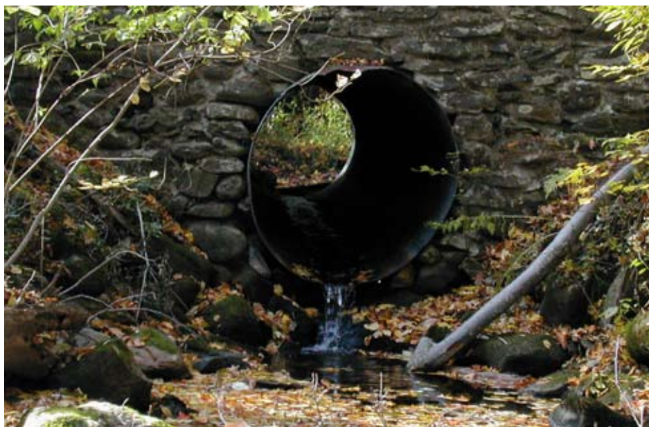
Figure 1.15—Many crossing structures are narrower than the stream and block fluvial processes that maintain aquatic habitats. The structures also impede aquatic species passage. Photo: Scott Jackson, University of Massachusetts.
