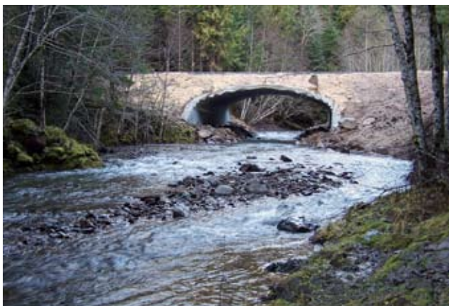
Figure 7.6—Multiplate open-bottom box.
