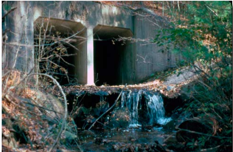
Figure 1.21—Outlet drop formed by scour at the downstream end of an asphalt apron. Photo: Scott Jackson, University of Massachusetts.
