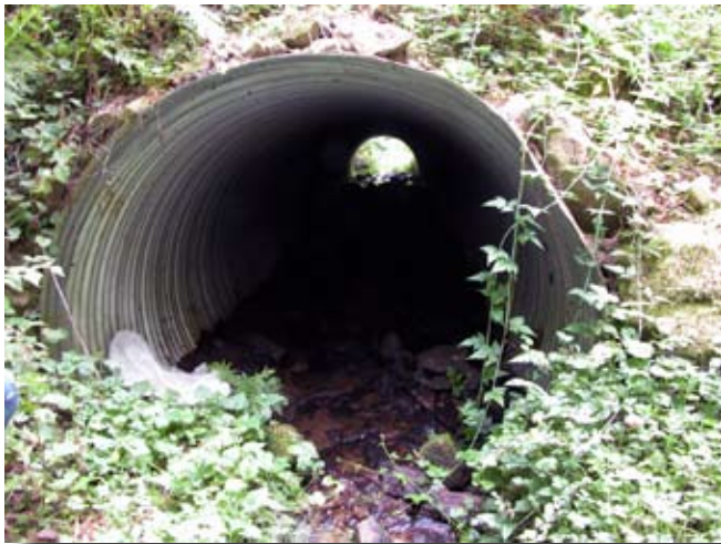
Figure 7.2—1-piece corrugated metal pipe (embedded).
