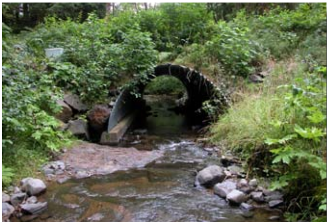
Figure 7.4—1-piece open-bottom arch.
