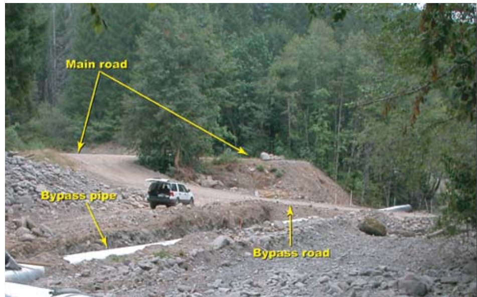
Figure 7.12—Typical construction site traffic bypass.
