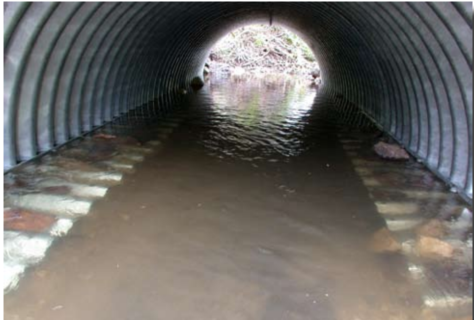
Figure 7.7—Open-bottom pipe arch with metal footings.
