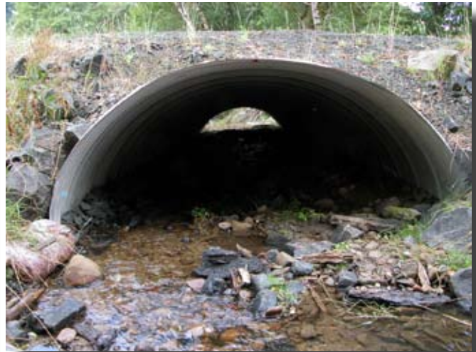
Figure 7.3—1-piece corrugated metal pipe arch (embedded).
