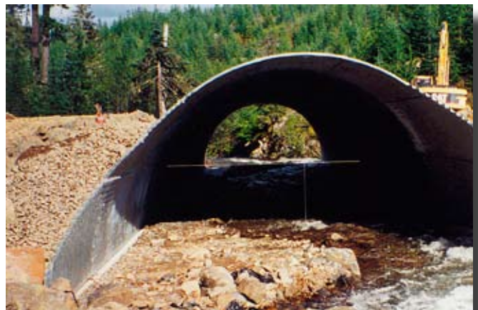
Figure 7.5—Multiplate open-bottom pipe arch.
