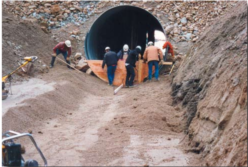
Figure 7.9—Shaping culvert bedding.
