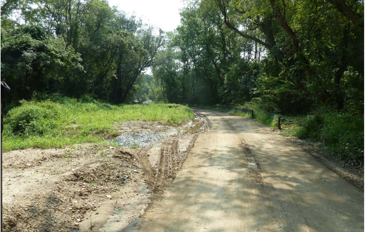
Photo 26. HR2. R.O.W. prior to restoration.
