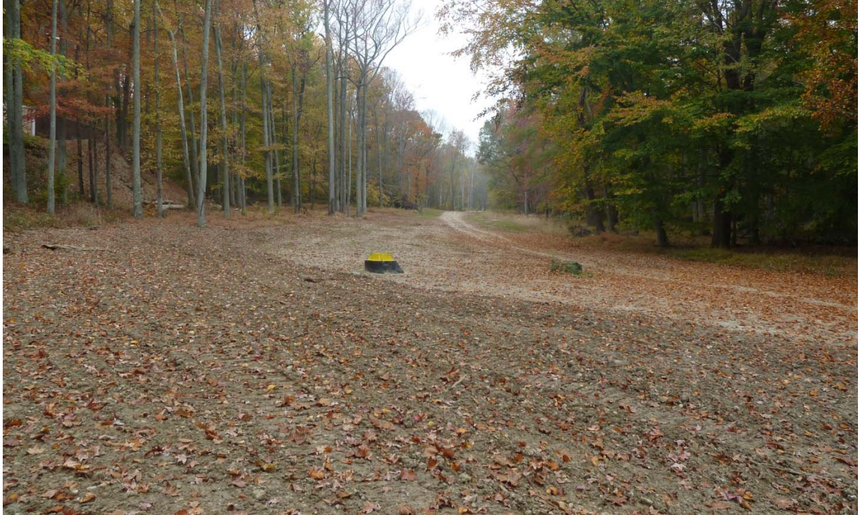
Photo 28. CHa and CHb. R.O.W. after leveling.
