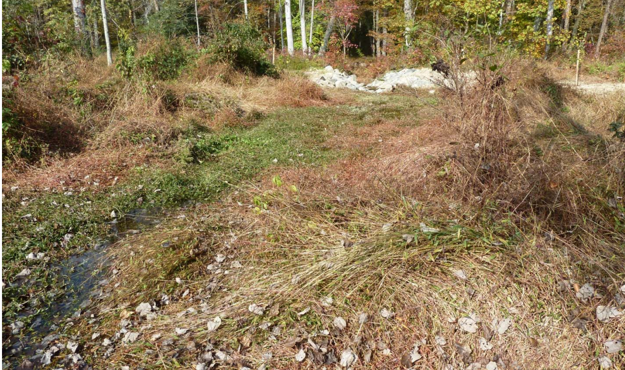
Photo 30. CHb. Stream flows through CHb and into CHa. Riprap used to stabilize the streambed where it crosses the R.O.W. is evident in the background.
