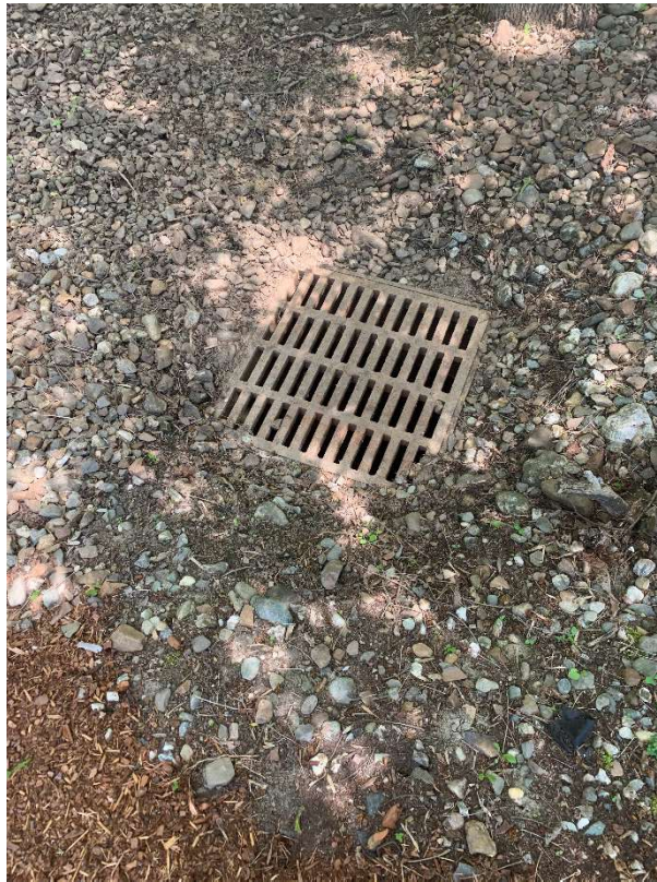
11. A storm drain that connects the ditch from photo 10.
