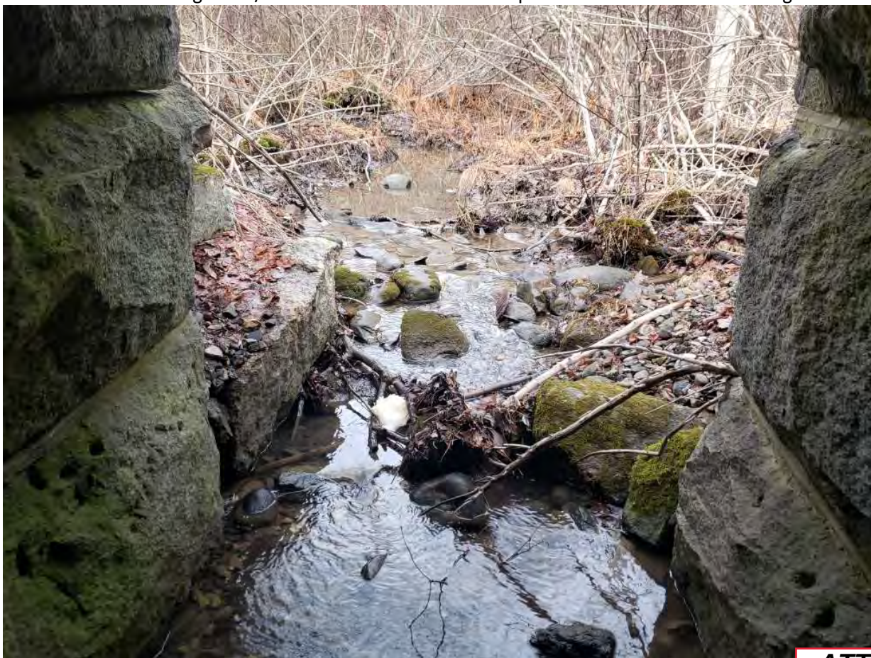
Photo 16: View looking west at inlet area of culvert beneath railroad.
