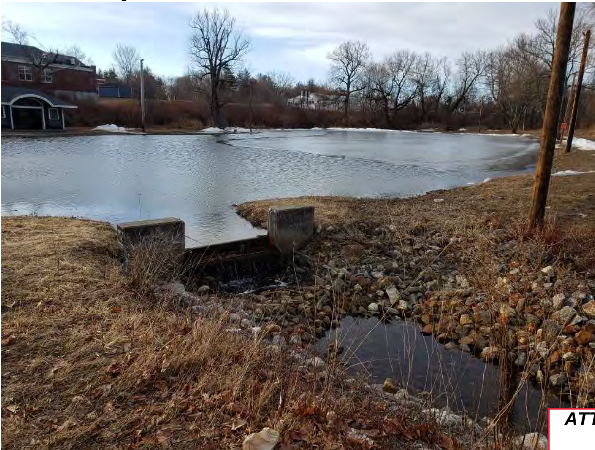
Photo 4: View looking south/southeast at water control structure near inlet of culvert beneath U.S. Route 1.
