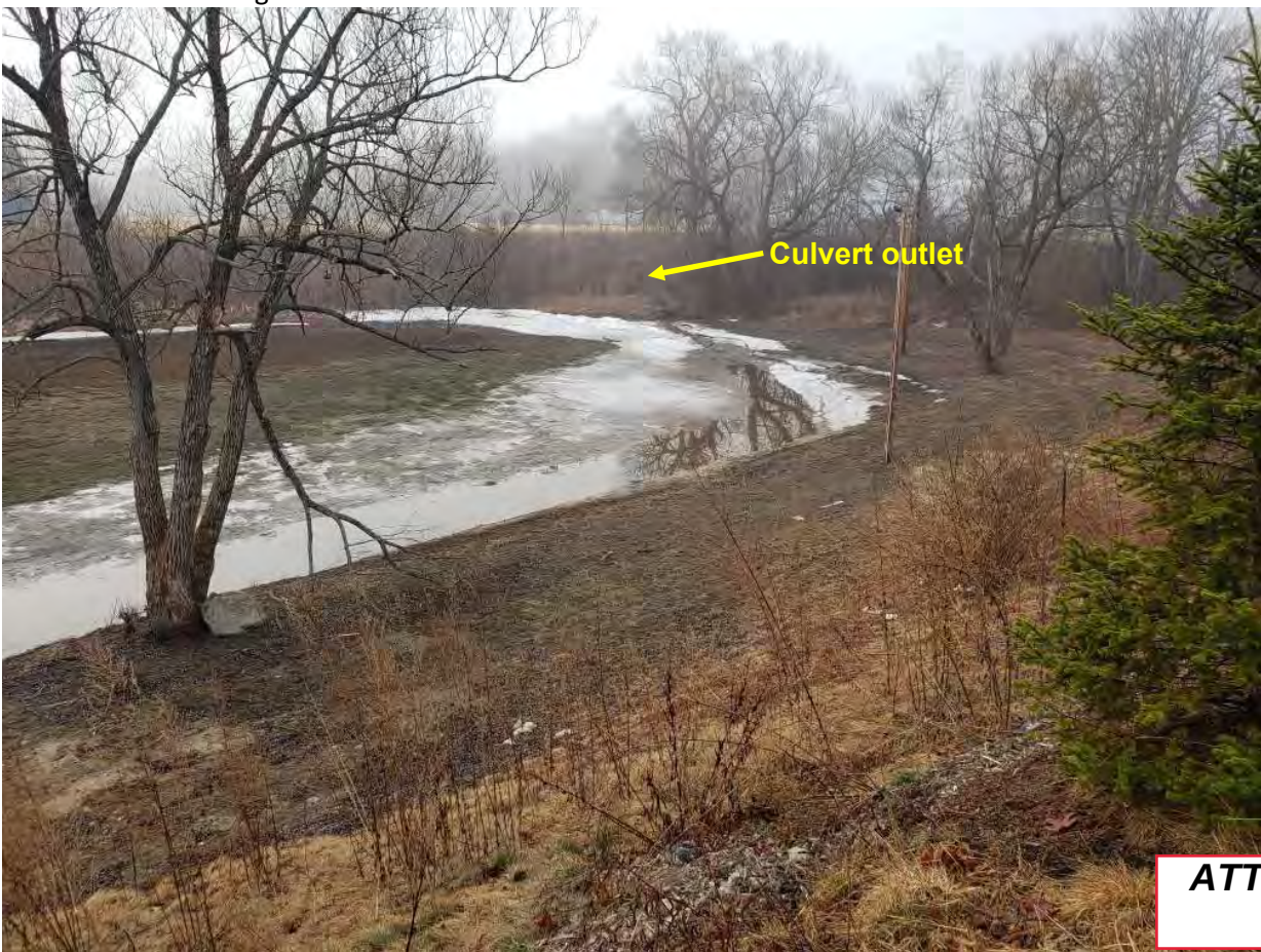
Photo 6: View looking southeast at channelized flow at toe of embankment; athletic field culvert in background.
