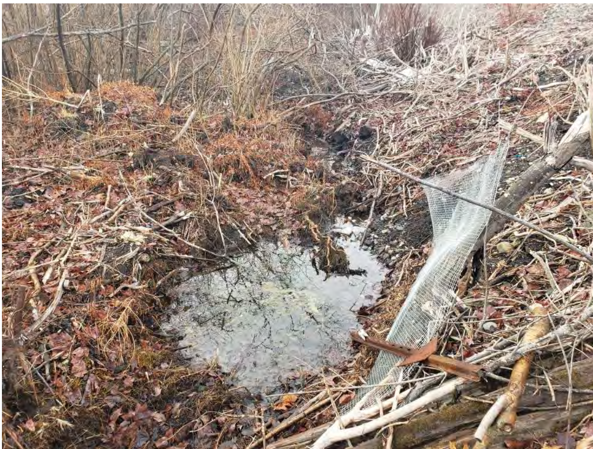
Photo 21: View looking at inlet area of 15-in. dia. clay pipe beneath railroad; subject AJD wetland in background.
