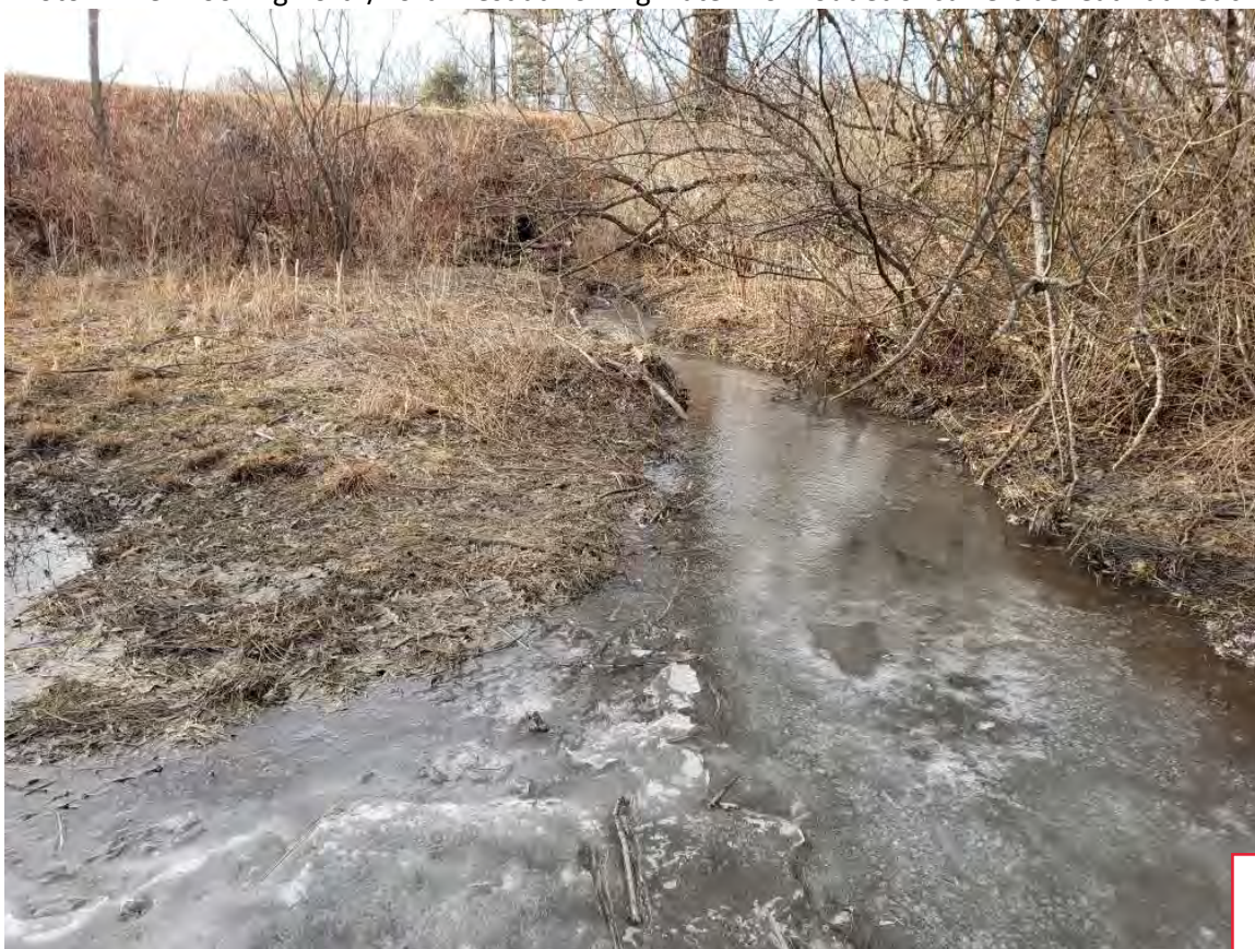
Photo 8: View looking south/southeast at flowing water from outlet of culvert beneath athletic field.
