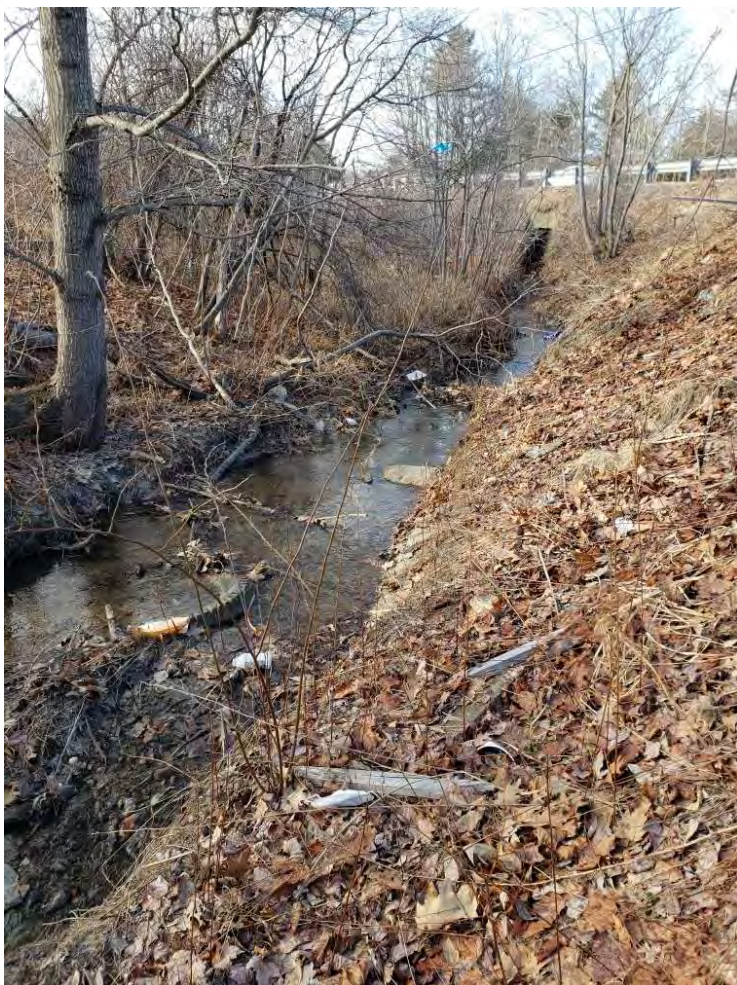
Photo 13: View looking southwest at outlet of box culvert beneath U.S. Route 1.
