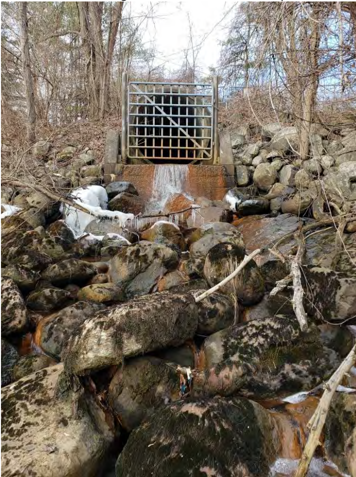
Photo 2: Looking southwest at outfall of "Brickyard Hollow" closed drainage.
