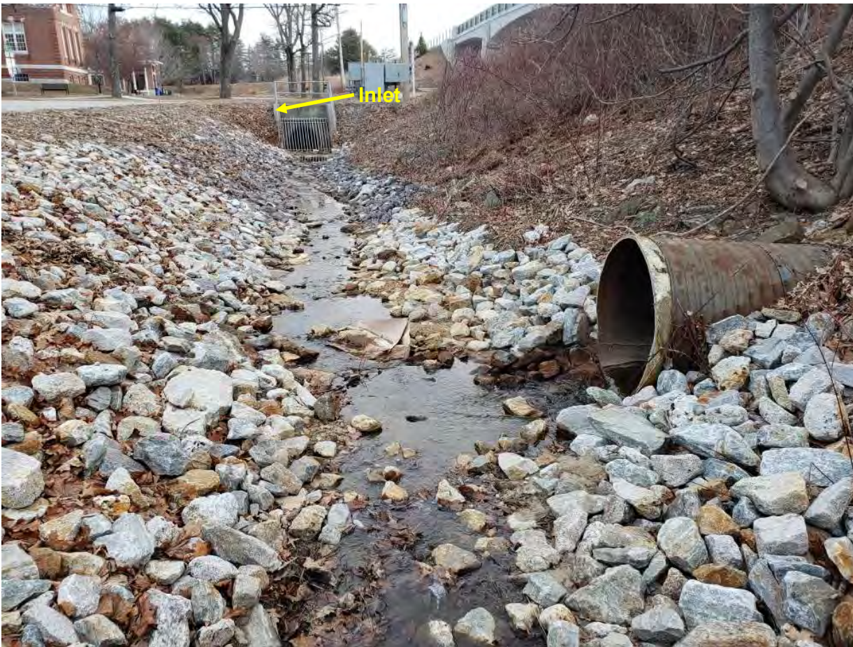
Photo 3: View looking northeast at outlet of culvert beneath U.S. Route 1 and towards inlet of closed drainage.
