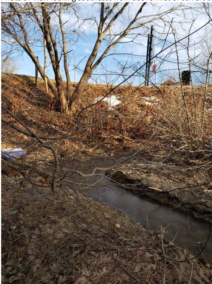
Photo 10: View looking northwest at inlet area of culvert beneath athletic field.
