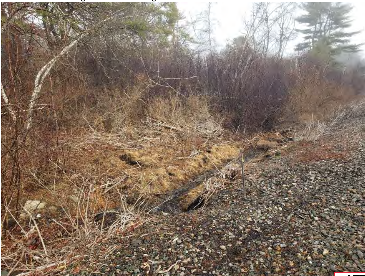
Photo 20: View looking at outlet area of 15-in. dia. clay pipe beneath railroad.
