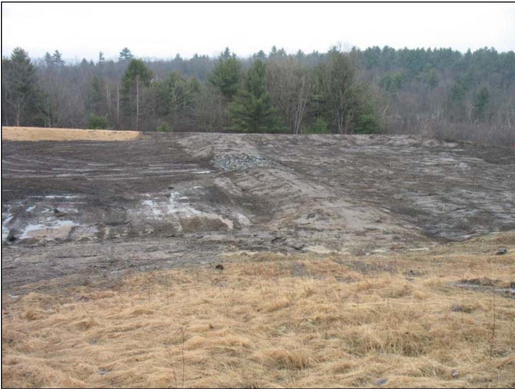
Photo 2. Facing south towards separator berm and spillway between upper two cells (28-Mar-2007.) Most of this berm will be removed in 2008/2009.
