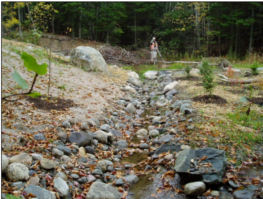
Photo 10. Restored stream channel at culvert removal location, looking upstream (east). Stantec, October 19, 2007.
