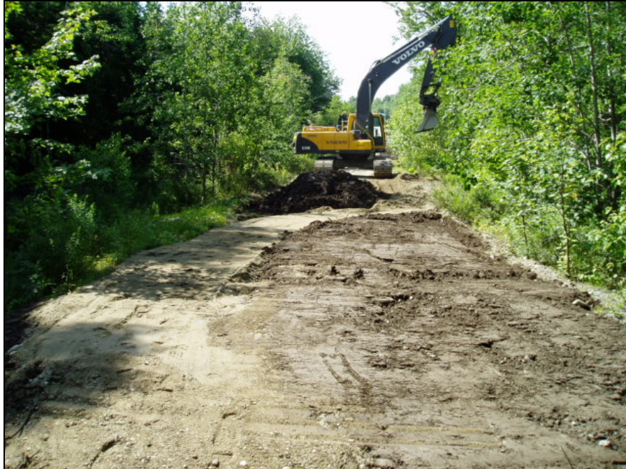
Photo 1. Excavator stripping gravel and adding topsoil in upland restoration area. Woodlot, July 25, 2007.
