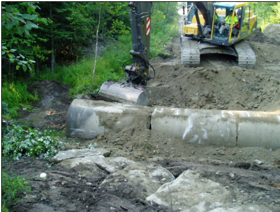
Photo 4. Removing 50-inch concrete culvert from wetland restoration area. Woodlot, July 25, 2007.
