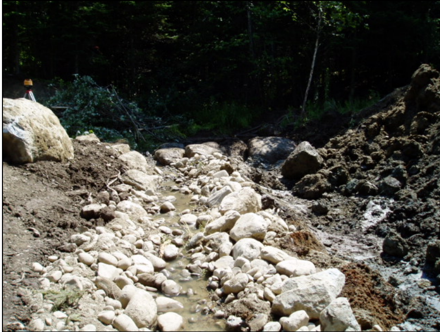
Photo 5. Re-established stream channel after culvert removal and placement of rocks, looking upstream (east). Woodlot, July 25, 2007.
