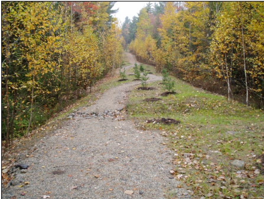
Photo 8. Water bar on sloped section of restored road. Also note trees already established along edges of old road. Stantec, October 19, 2007.
