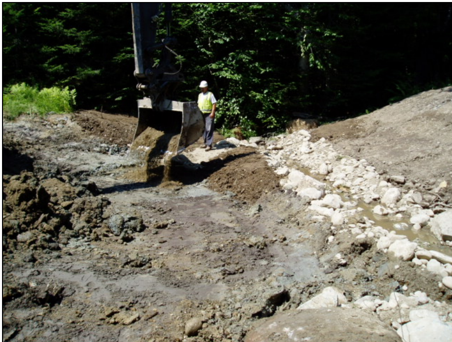
Photo 6. Adding topsoil to wetland restoration area, looking west (downstream). Re-established channel where culvert was is shown on right. Woodlot, July 25, 2007.
