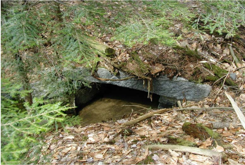
Granite culvert at Station 2+340 L
