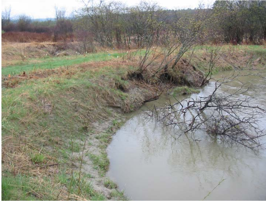
Photo 9. View upstream of lower section of streambank stabilization area showing bank scarring that resulted when large shrub clump located between two stabilization areas slid into river in 2004-2005. 5-3-06.
