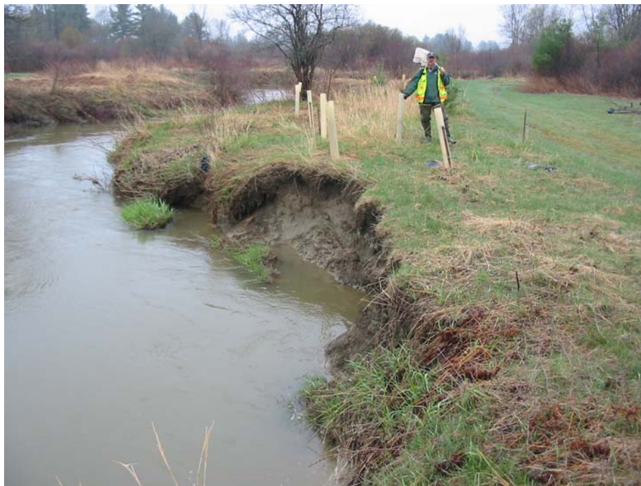
Photo 6. View of bank erosion near plant group 2 that occurred over the winter of 2005-2006. 5-3-06.
