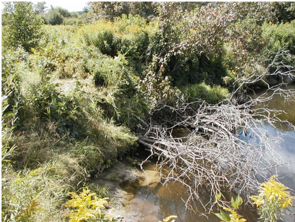
Photo 18. Downstream section of streambank stabilization area at the end of the third growing season showing vegetation regrowth around shrub clump that slumped previously. 8-24-06.
