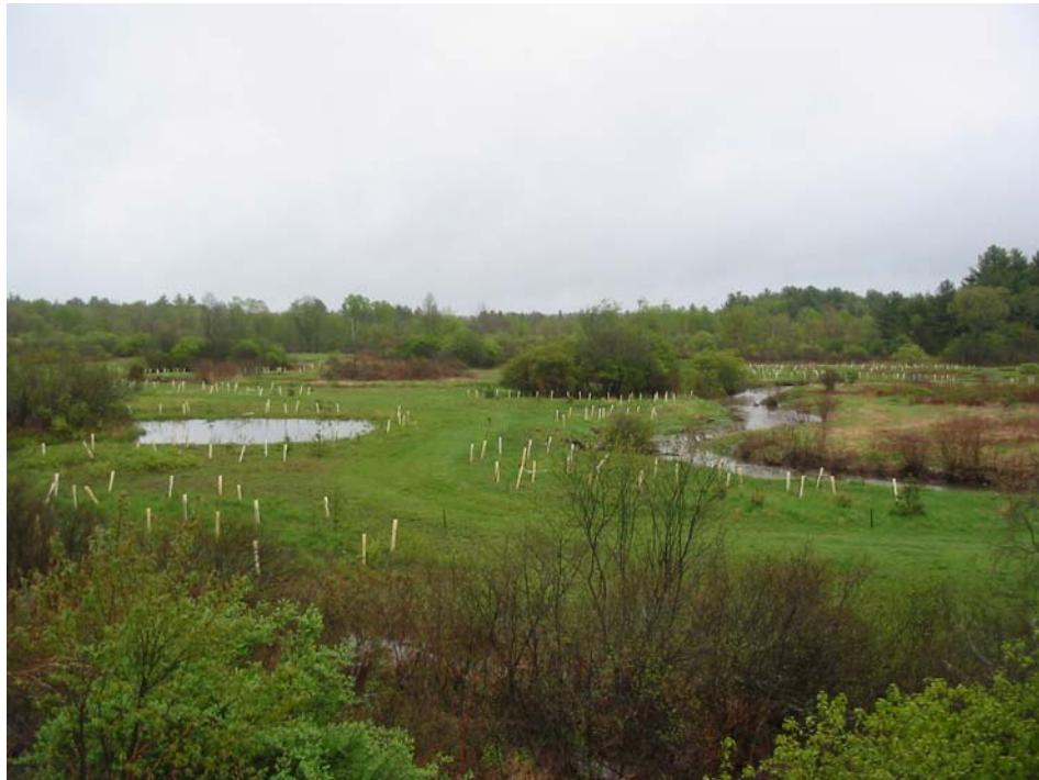
Photo 4. View of floodplain enhancement area at Royal River site from railroad embankment showing plant groups, shallow pool, and channel. 5-16-06.
