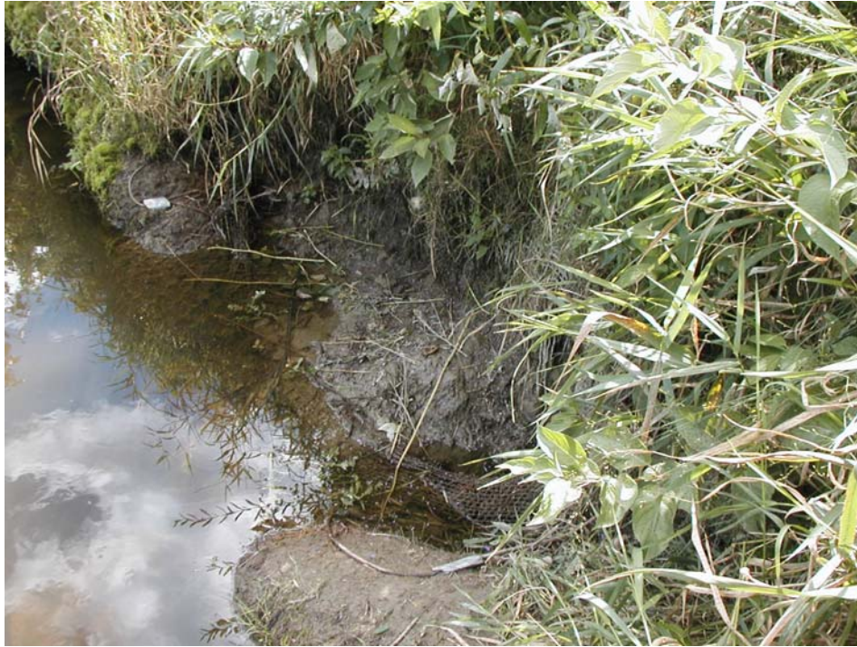
Photo 17. Close up of slump in coir log at toe as a result of beaver activity in middle section of streambank stabilization area. 8-24-06.
