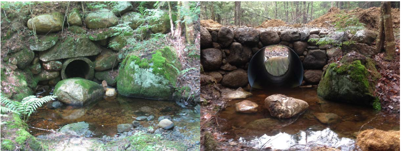
Avery Brook Woods Road culvert replacement project before and after – Francestown, NH
