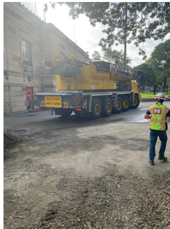
John Rudd on the job at the Muddy River Flood Reduction Project.
