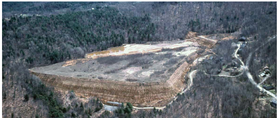
Elizabeth Mine Tailing Pile (pre-construction) looking south, May 2003.
