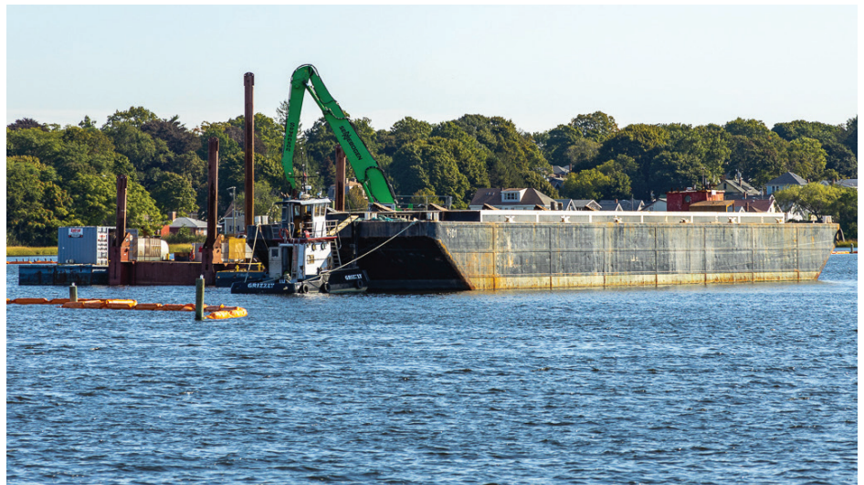
A dredge performs work in New Bedford Harbor.
