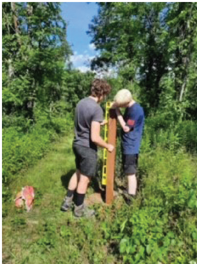
Leveling the sign post before installing the sign.
