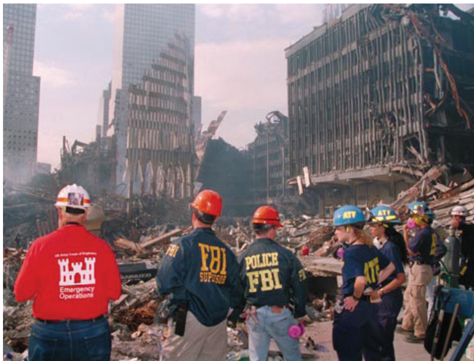
A USACE Team member, FBI and ATF personnel observe the remnants of the World Trade Center. Photo by F:T:Eyre
