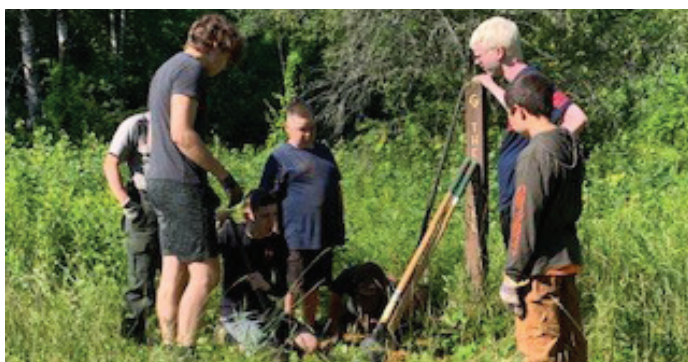
Tyler Kulacz (left) and volunteers digging to install post for sign.
