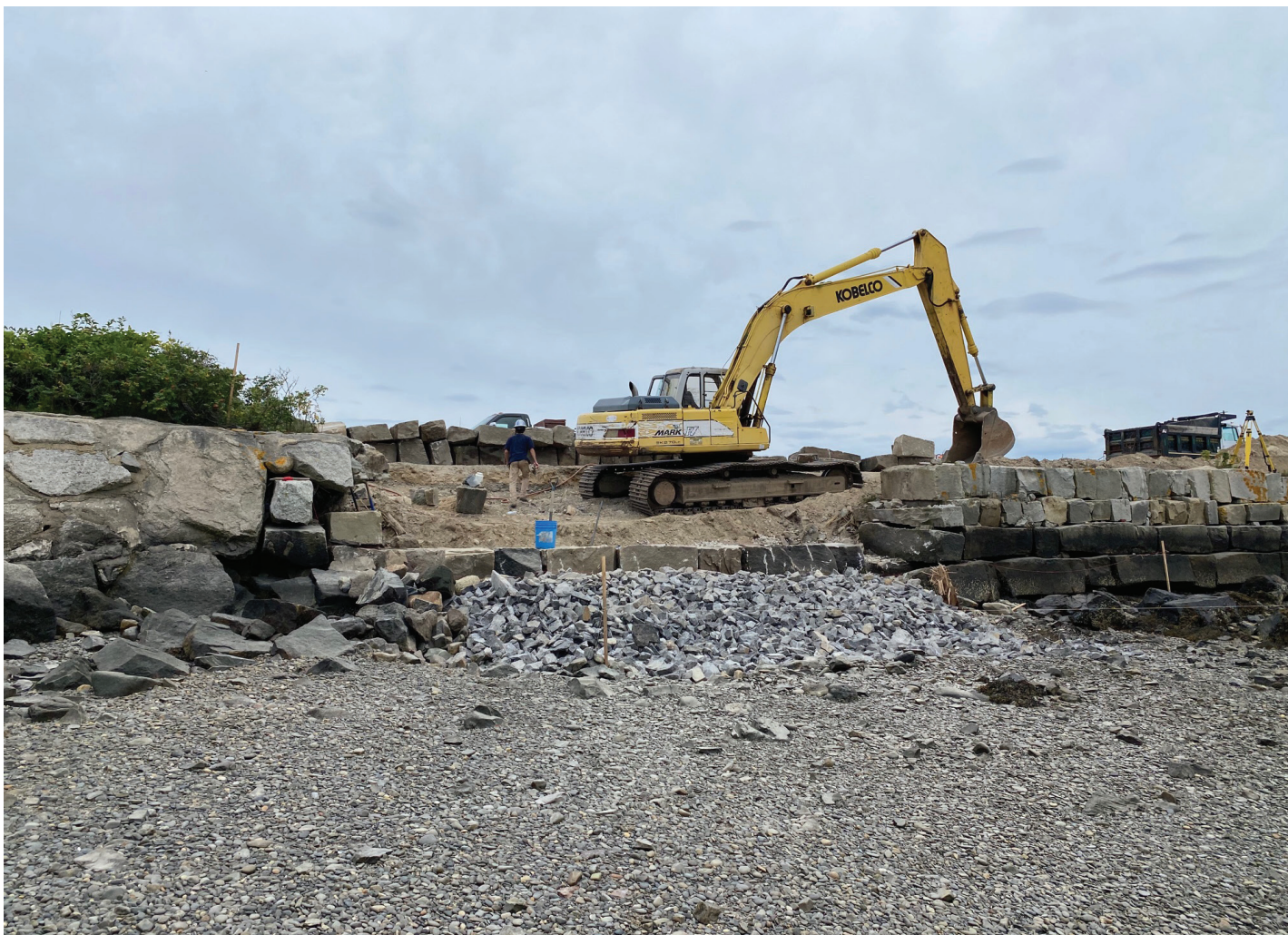
Mohawk, Northeast, Inc. performs repair work at Kennebunk, Maine
