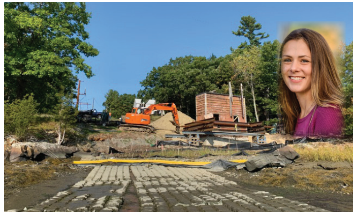
Historic cable house moved and being restored. Inset: Lindsey Lefebvre.
