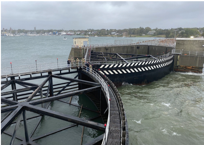
Brig. Gen. Thomas Tickner sees the New Bedford Hurricane Barrier operate during his visit to the project.
