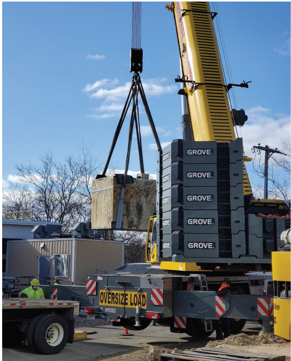
Crane lifting the WBC to the building opening. Note some of the counterweights on the back of the crane – a total of 297,600 pound was needed to ensure a safe lift.
