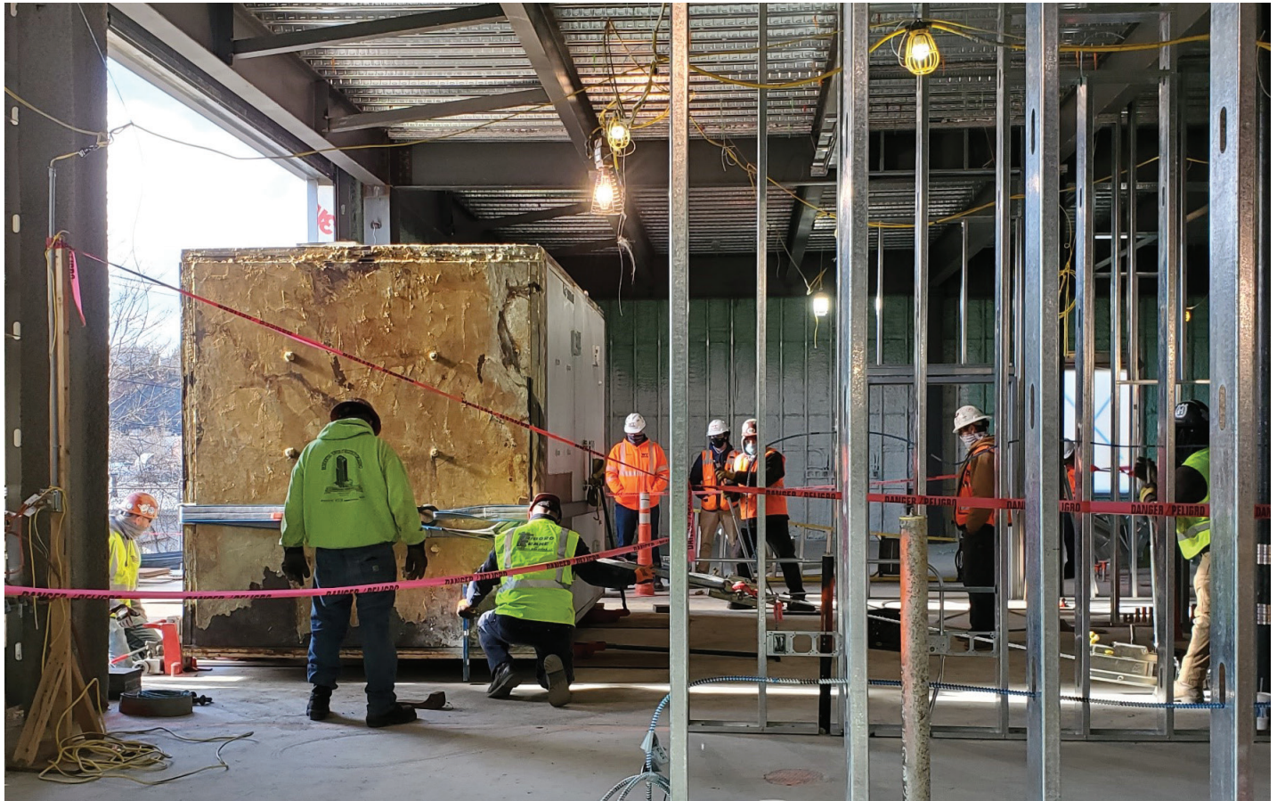
Adjusting the WBC to its final location within the building.
