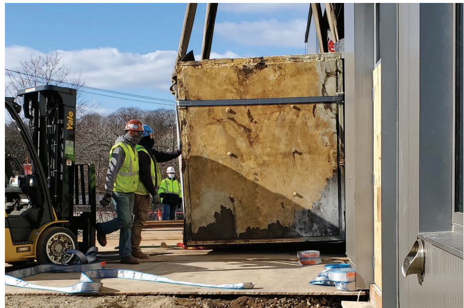
WBC at new building opening – set on top of rollers to guide the structure into the building.
