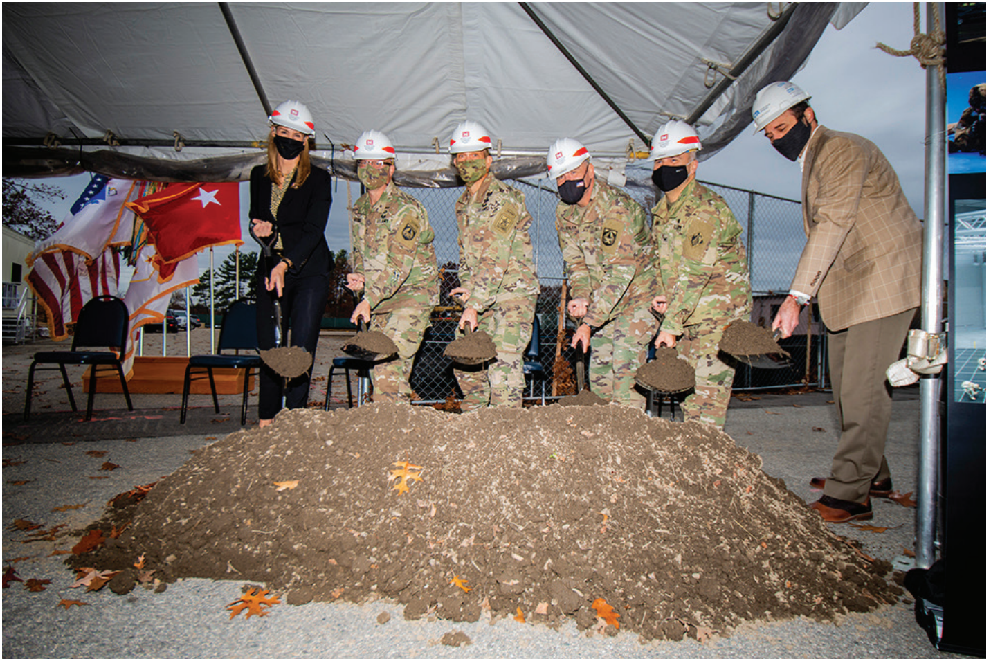
Members of the official party break ground on the S2PRINT facility.
