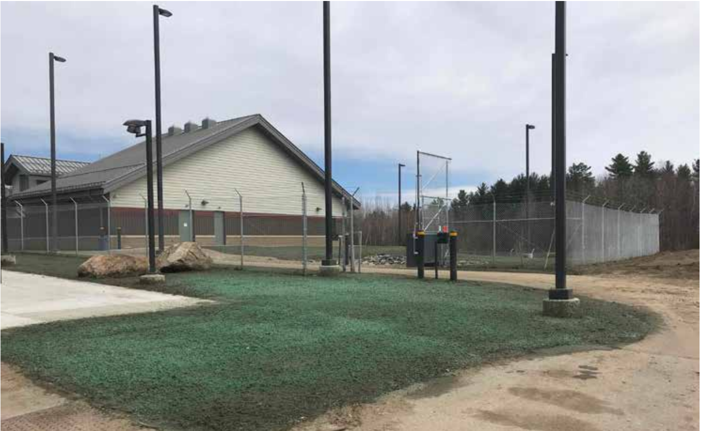
The New England District team completed Border Patrol facility in Swanton, Vermont, April 9.
