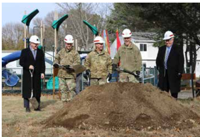
Col. William Conde (center) joins Brig. Gen. Vincent Malone (second from right) and other officials in breaking ground for the Natick Family Housing project.
