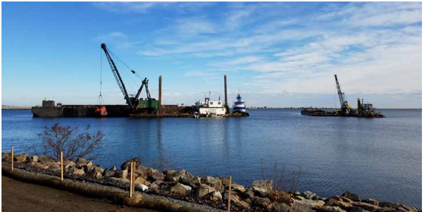
Dredging to remove shoals from the Plymouth Harbor federal navigation project is underway.
