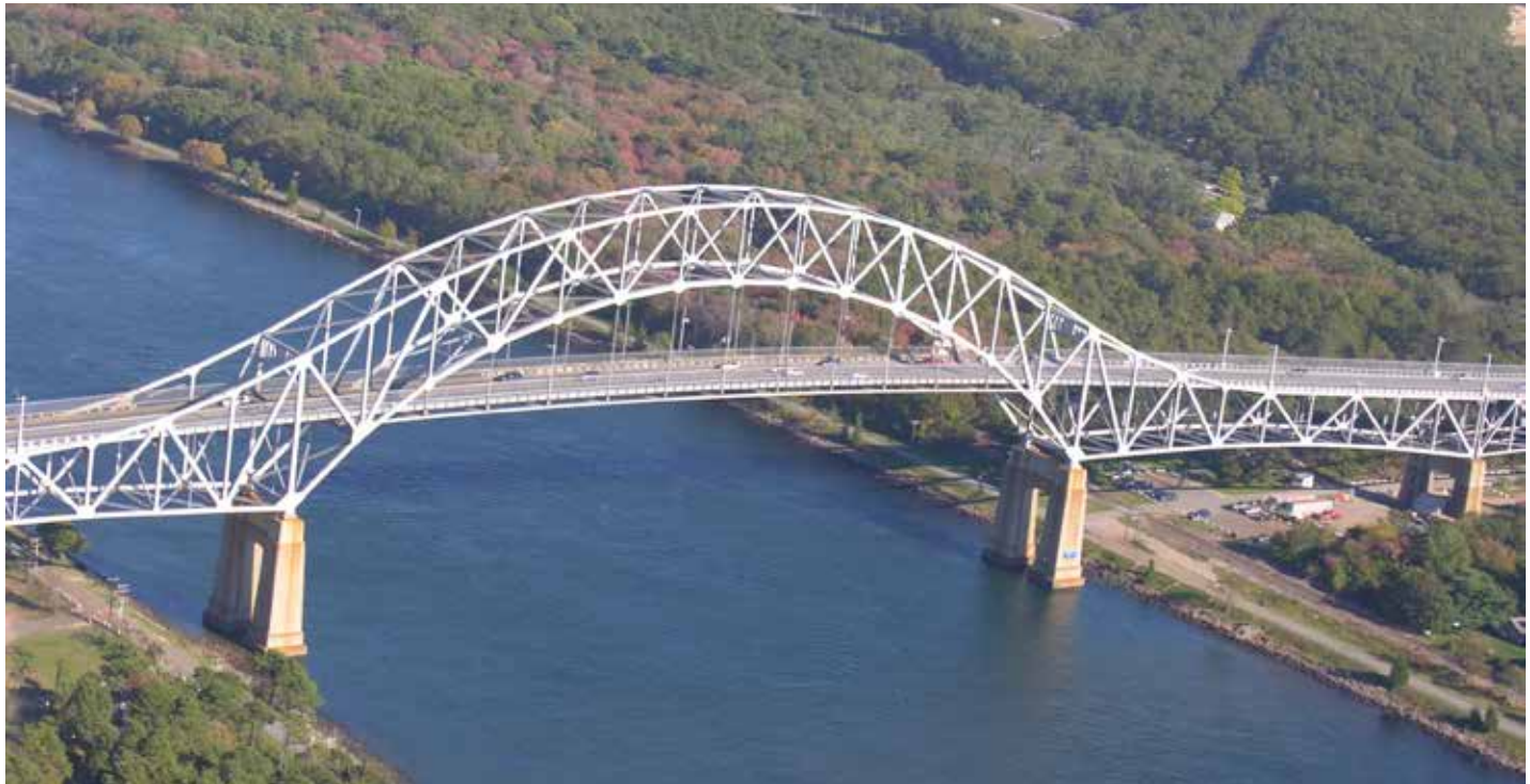
Repairs on the Bourne Bridge are set to begin in March or April.
