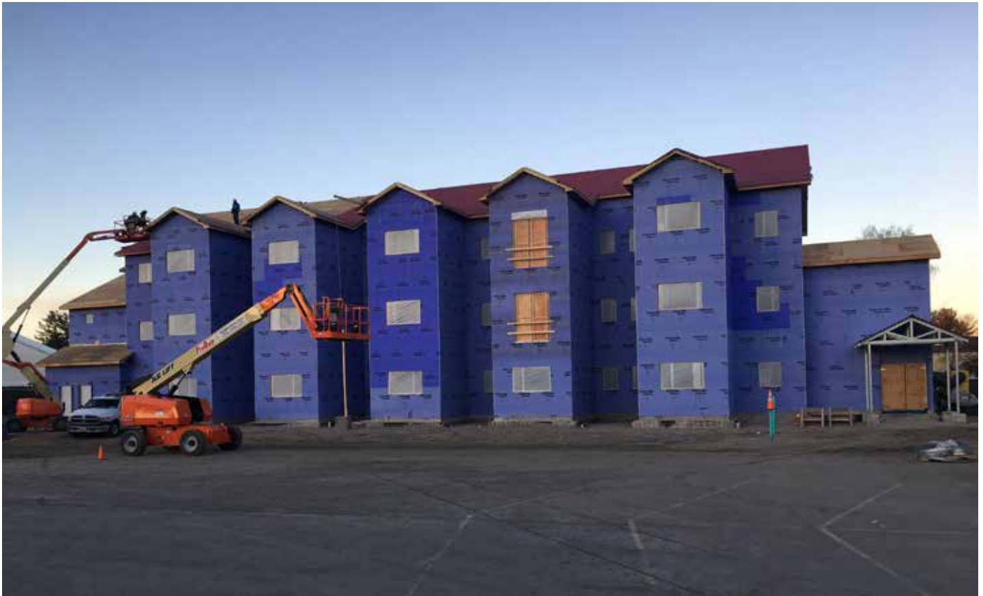
Hanscom Dormitory was weather tight before the winter set in.
