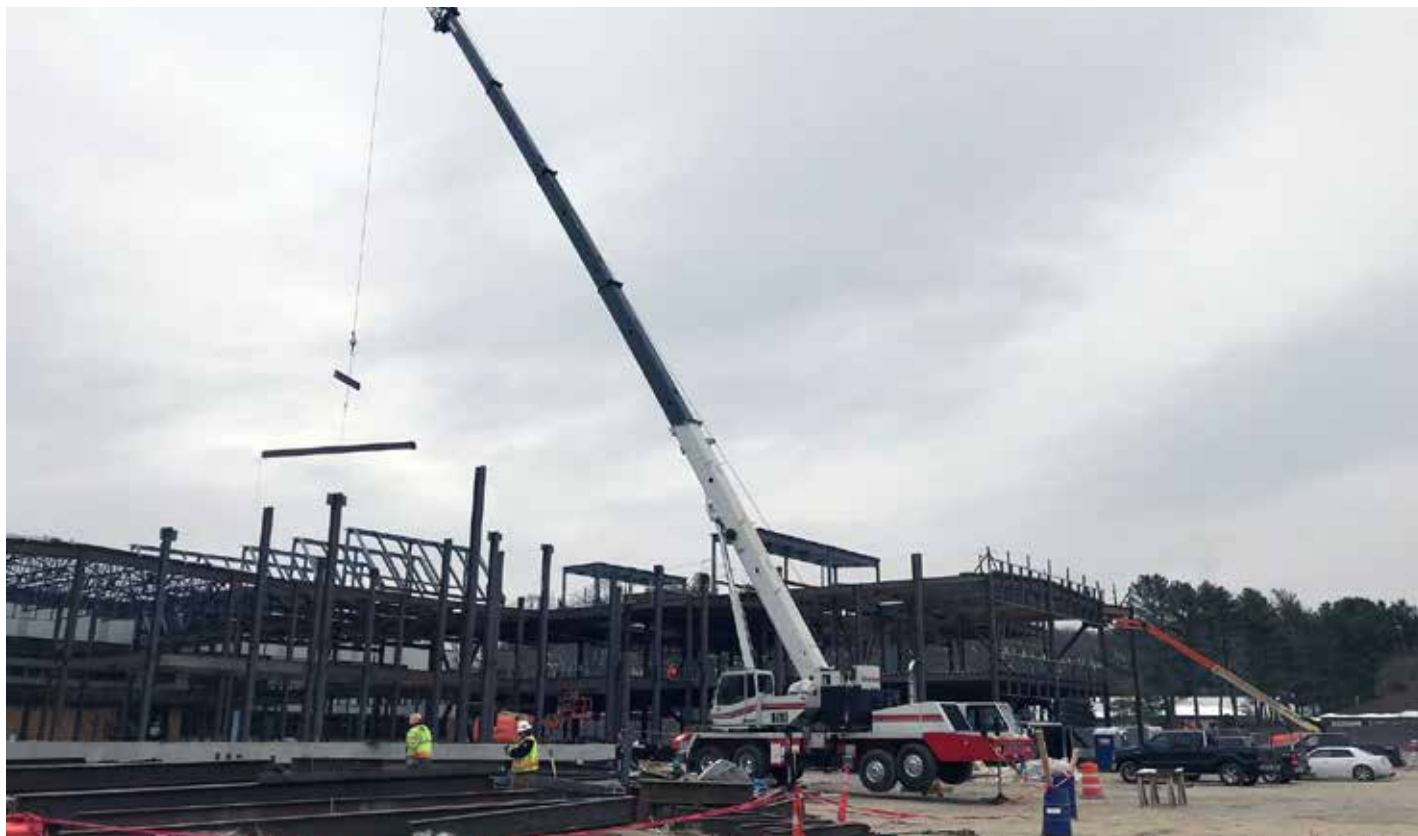
The Hanscom Air Force Base Primary School is under construction.
