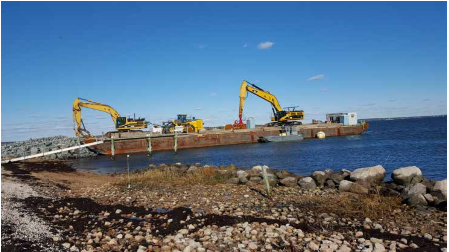
Final preparation of restoration on Bird Island.
