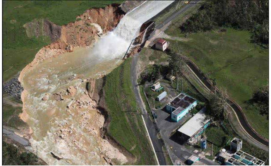
An aerial view of the Guajataca Dam in Puerto Rico.
