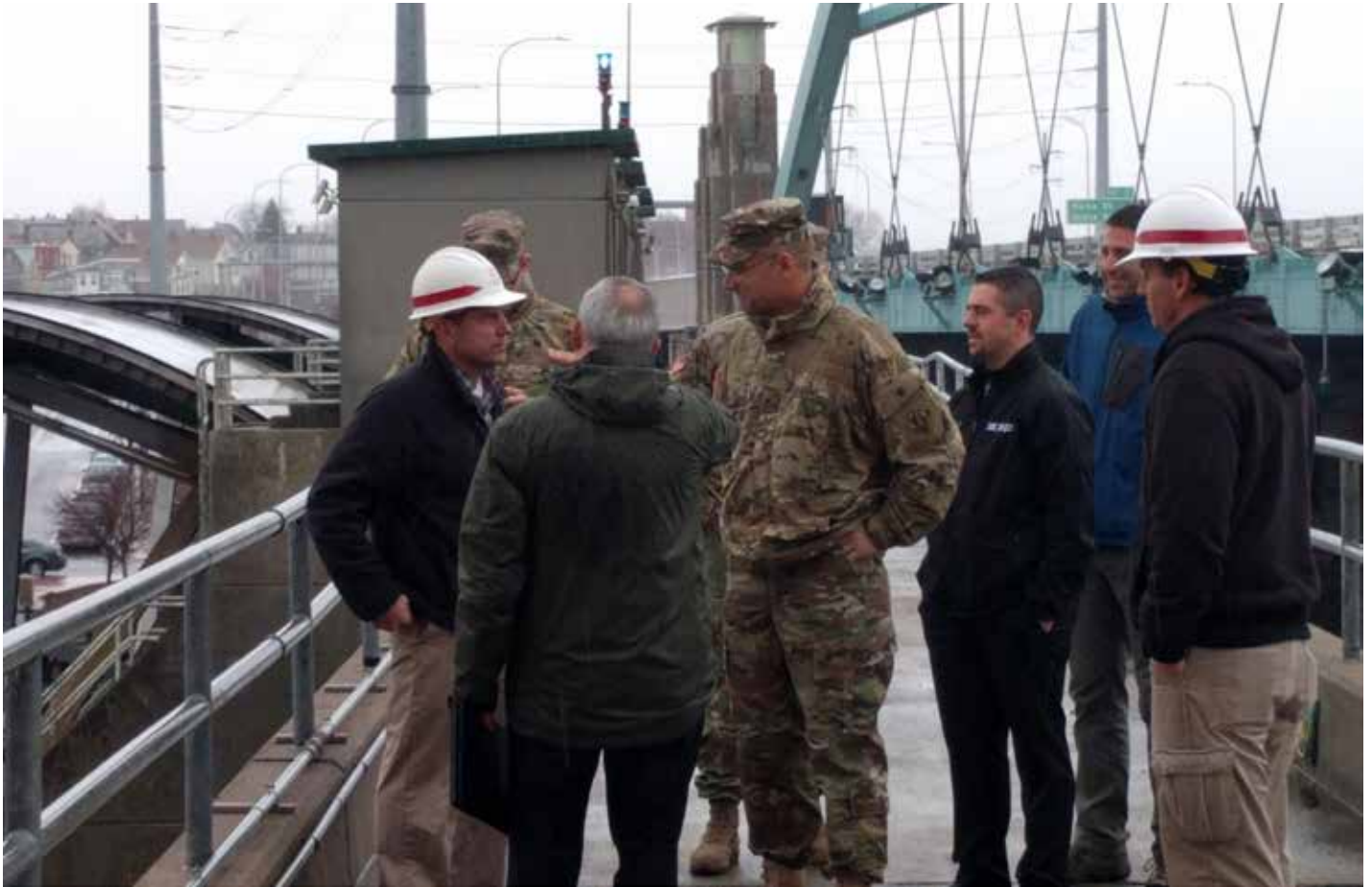
Brig. Gen. William Graham, North Atlantic Division Commander gets a tour and briefing of the Fox Point Hurricane Barrier in Providence, Rhode Island.
