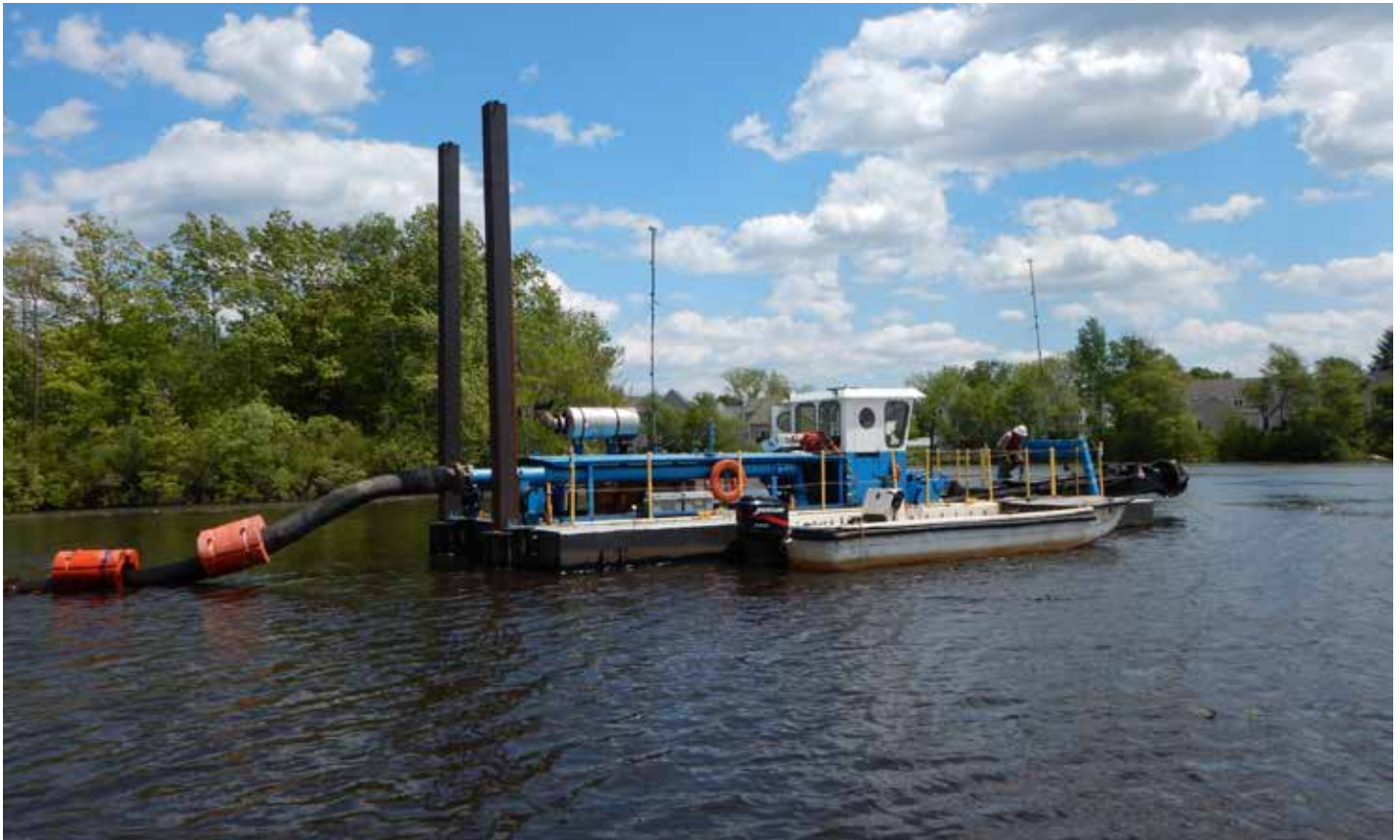
Dredging Milford Pond was key to restoration efforts.
