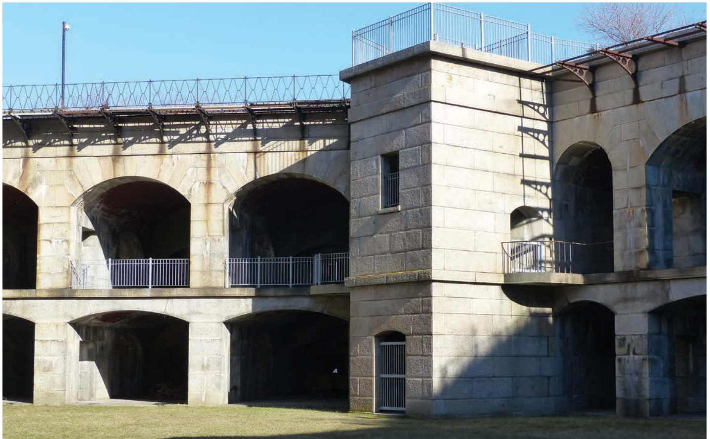
The New England District and Tantara Associated Corporation installed fall protection barricade railings all over Fort Rodman.
