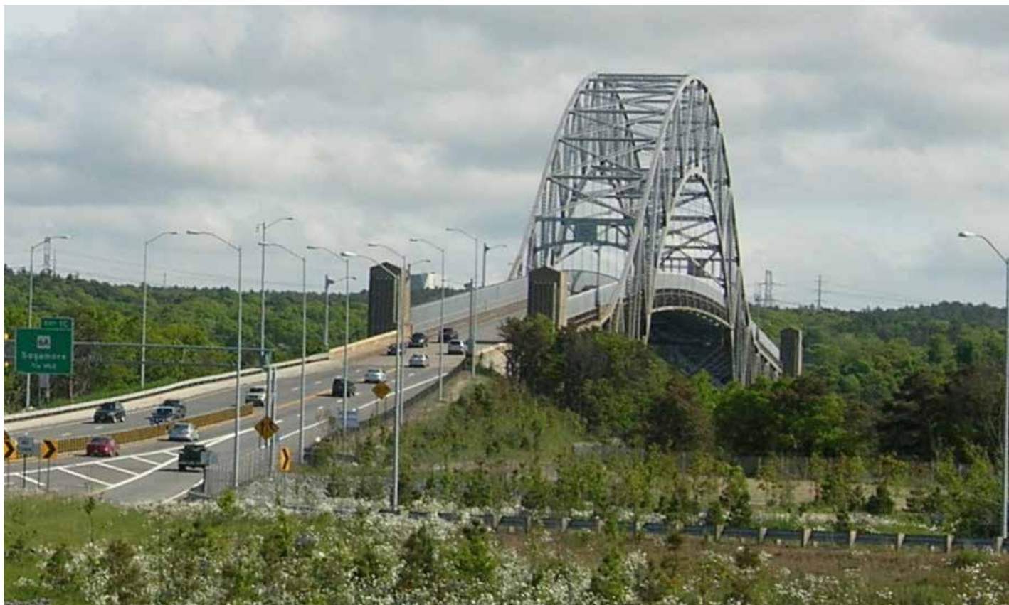
Lane restrictions have begun on the Cape Cod Canal's Sagamore Bridge.
