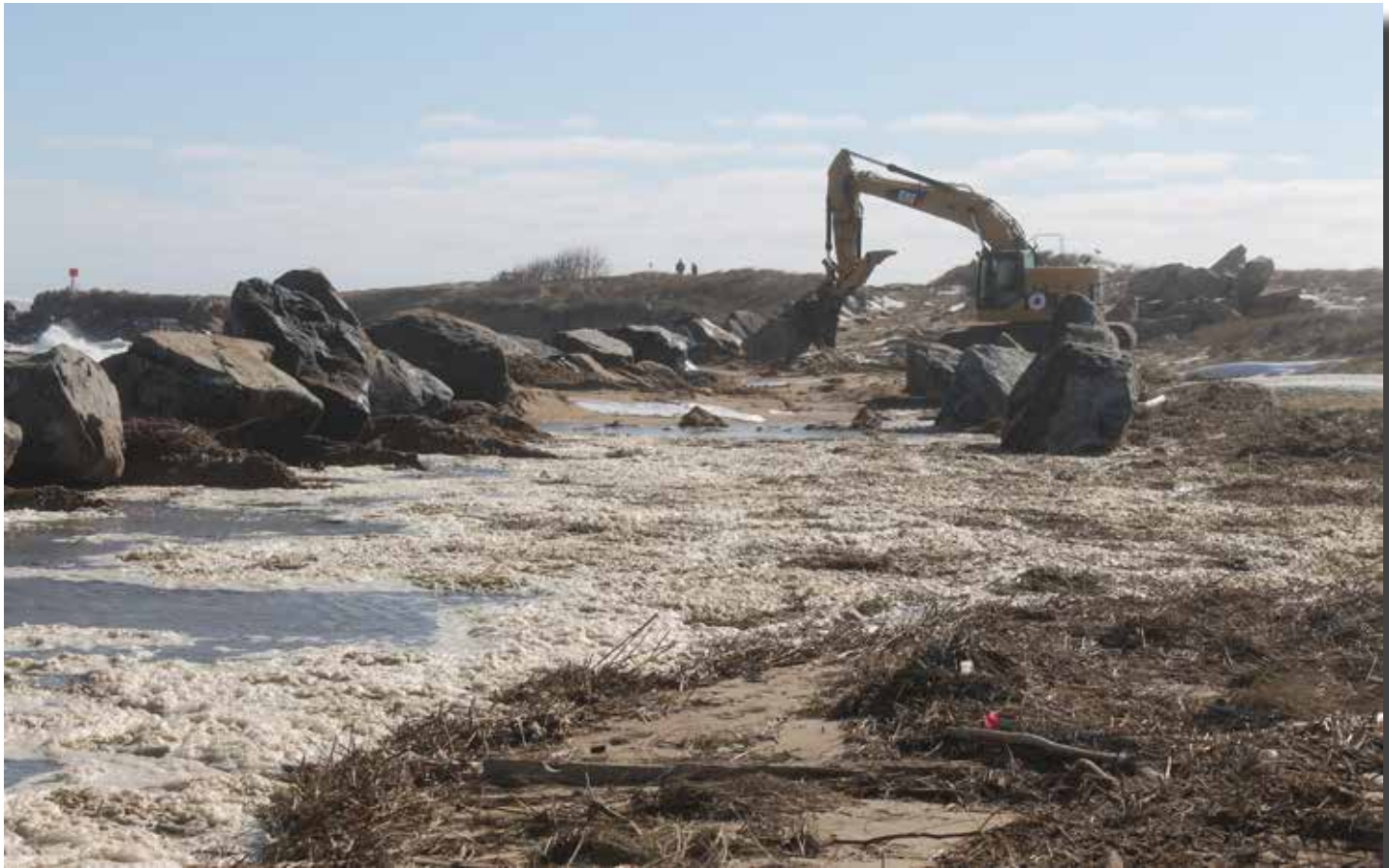
Work being performed on the Newburyport South Jetty in Newburyport, Mass.
