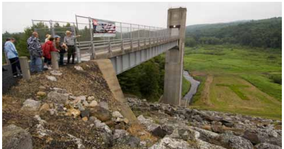
Thomaston Dam in Connecticut.
