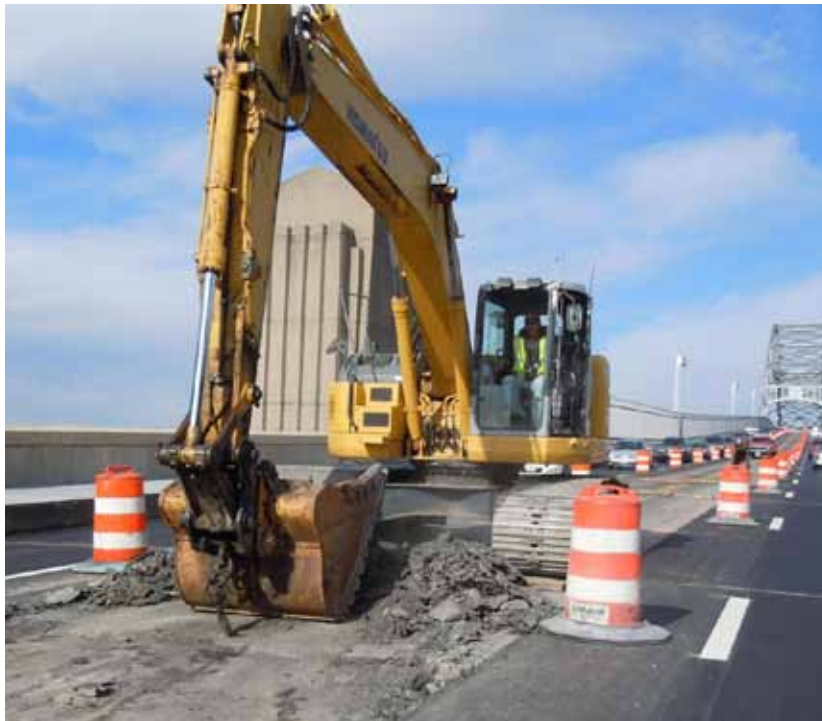
Repair work performed on the Bourne Bridge in 2010.
