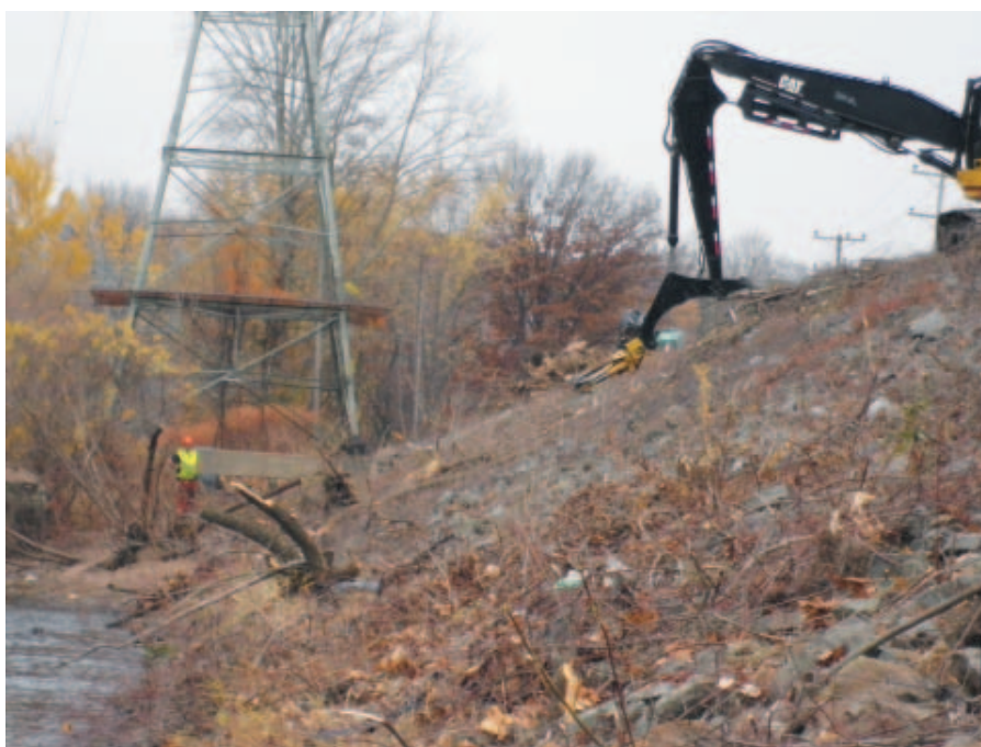
Heavy equipment operated by contractor J. Cook, Inc., of Upton, Mass., pulls a root ball from the "toe" of the Social District Levee. (Photo by Joe Zanca)
