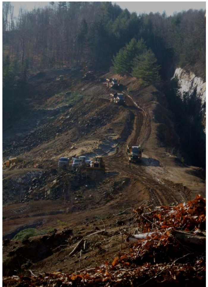
Work at the Elizabeth Mines in Maine is progressing.
