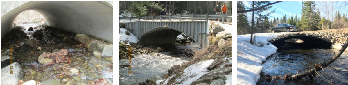
Figure 3-8. Culvert Replacement Projects in Northern Maine Utilizing a 1.2x Bankfull Width Approach and “Stream Simulation” Design Principles
