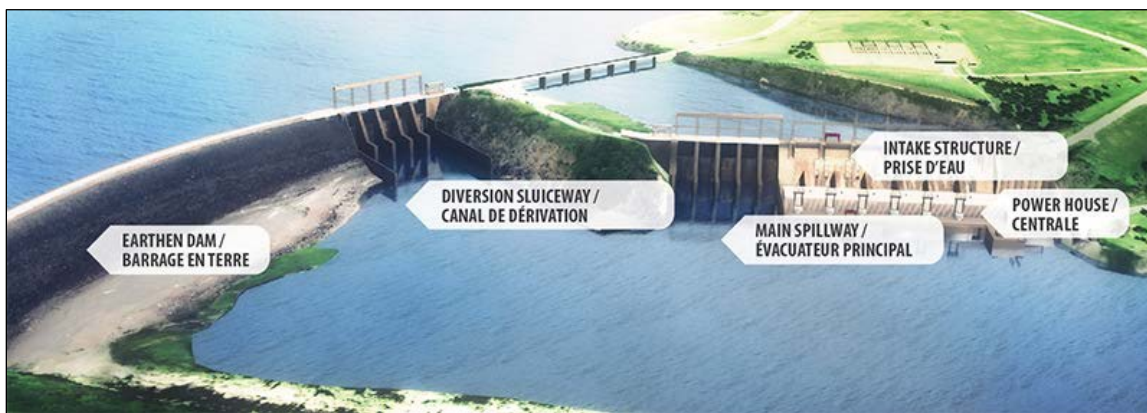
Figure 3-10. Schematic Representation of the Existing Mactaquac Dam
