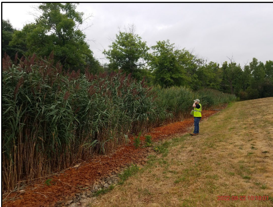
Photograph 18. Dense phragmites growth along eastern unmaintained drainage swale (22 August 2022).
