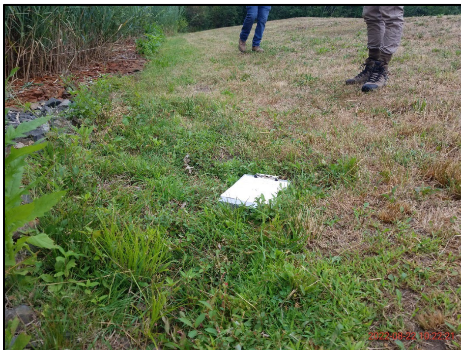
Photograph 8. Slight depression in the grass cover of the soil cap adjacent to the eastern drainage swale (22 August 2022).
