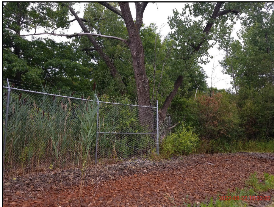
Photograph 3. Southern swale looking south; large tree growing through perimeter fence (22 August 2022).
