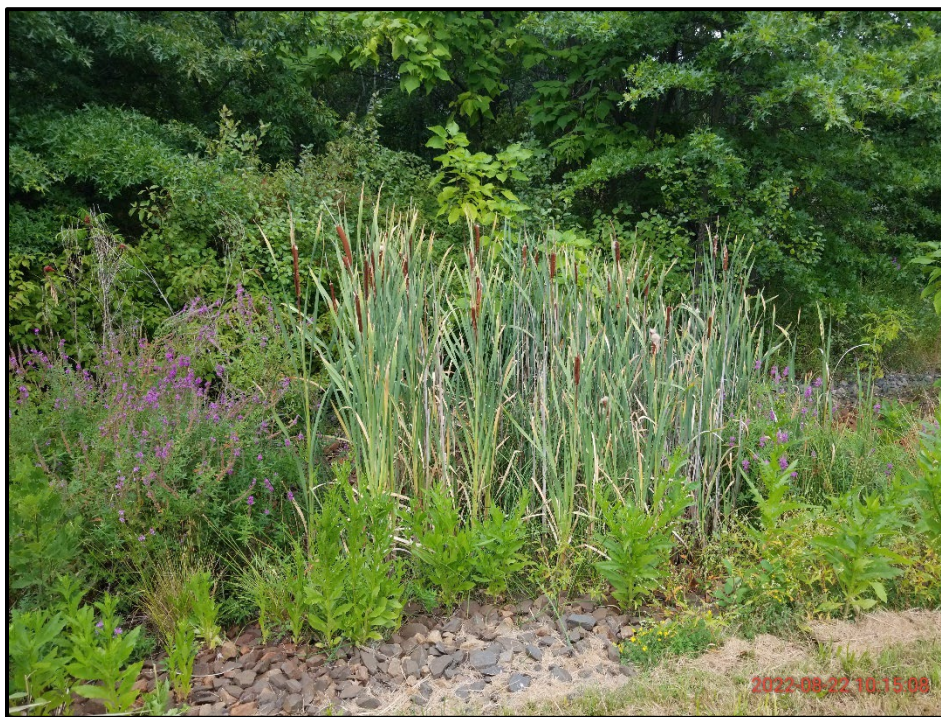
Photograph 14. Northern drainage swale looking northeast showing vegetation growth in swale (22 August 2022)
