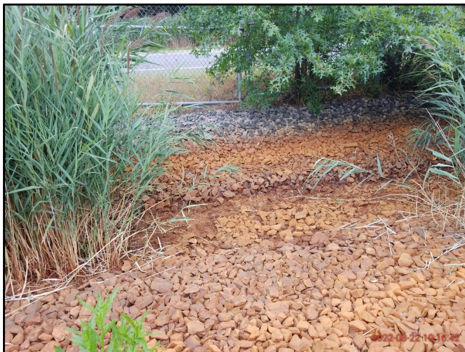
Photograph 16. Phragmites growth in drainage swale and tree growth blocking exterior of northeastern gate adjacent to Greenough Boulevard. (22 August 2022).
