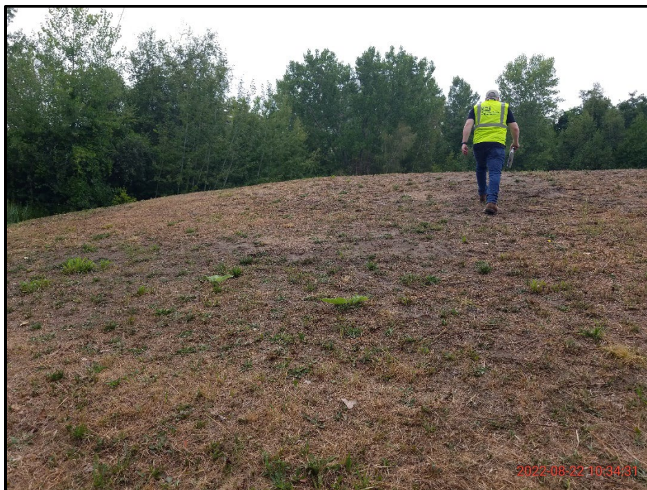
Photograph 10. Bare patches near crest of southern section (looking northwest) of the soil cap (22 August 2022).
