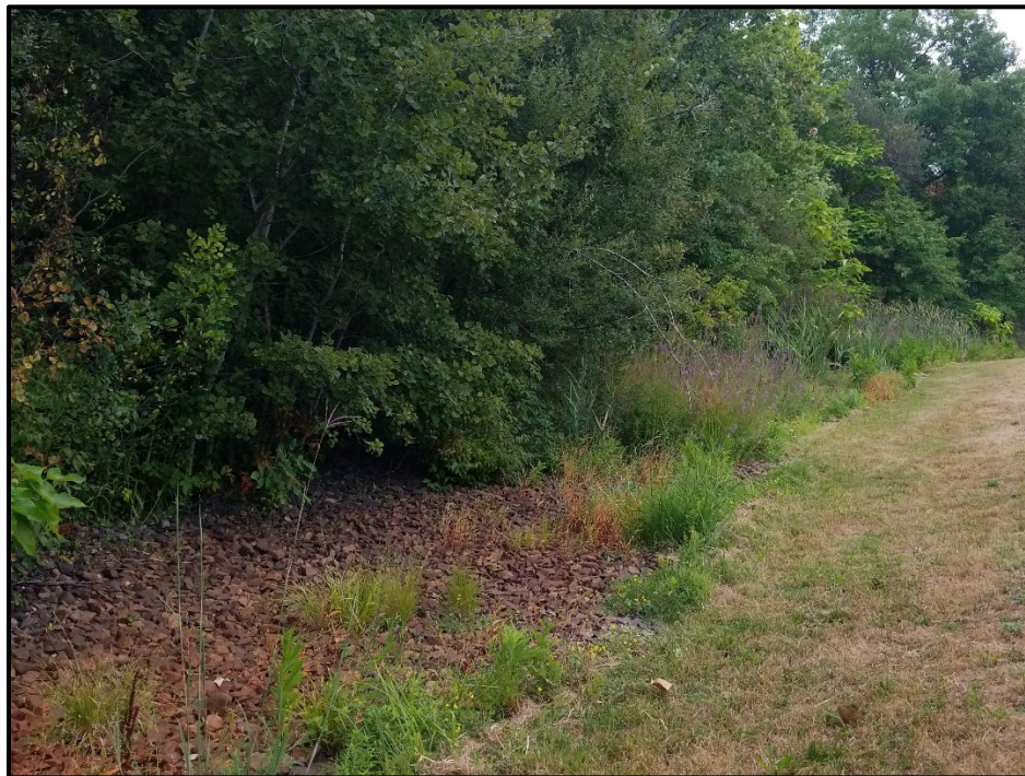
Photograph 15. Northern drainage swale with dense vegetation growth looking southwest towards Greenough Boulevard (22 August 2022)
