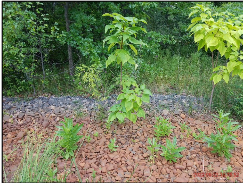
Photograph 13. Northern drainage swale showing woody vegetation growth in swale riprap (22 August 2022)
