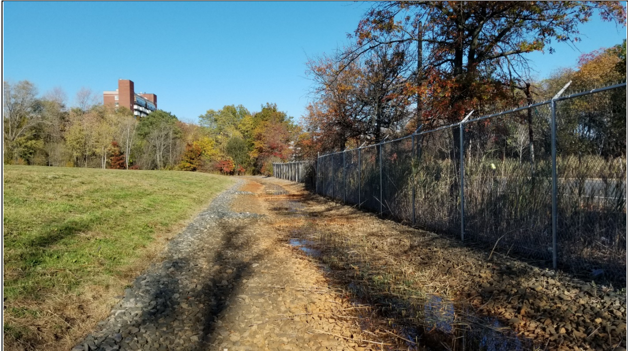
Photo 5. Drainage ditch looking northeast/upstream of the surface water discharge grate on the eastern swale (Photo 6 below). Note brown iron staining and Phragmites stubble (to be treated with herbicide). Greenough Boulevard is to the right.
