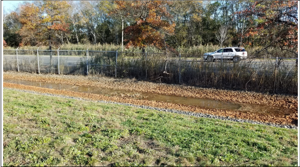
Photo 7. Upper portion of eastern swale parallel to Greenough Boulevard, showing ponded water, iron staining on the riprap/channel armor, and Phragmites stubble.
