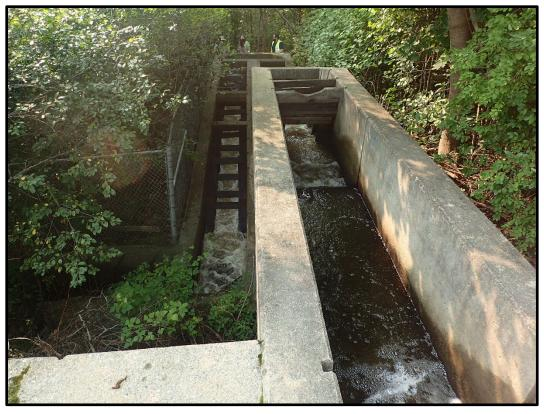
Figure 8: Denil-type Fish Ladder near the East Elm Street Dam
