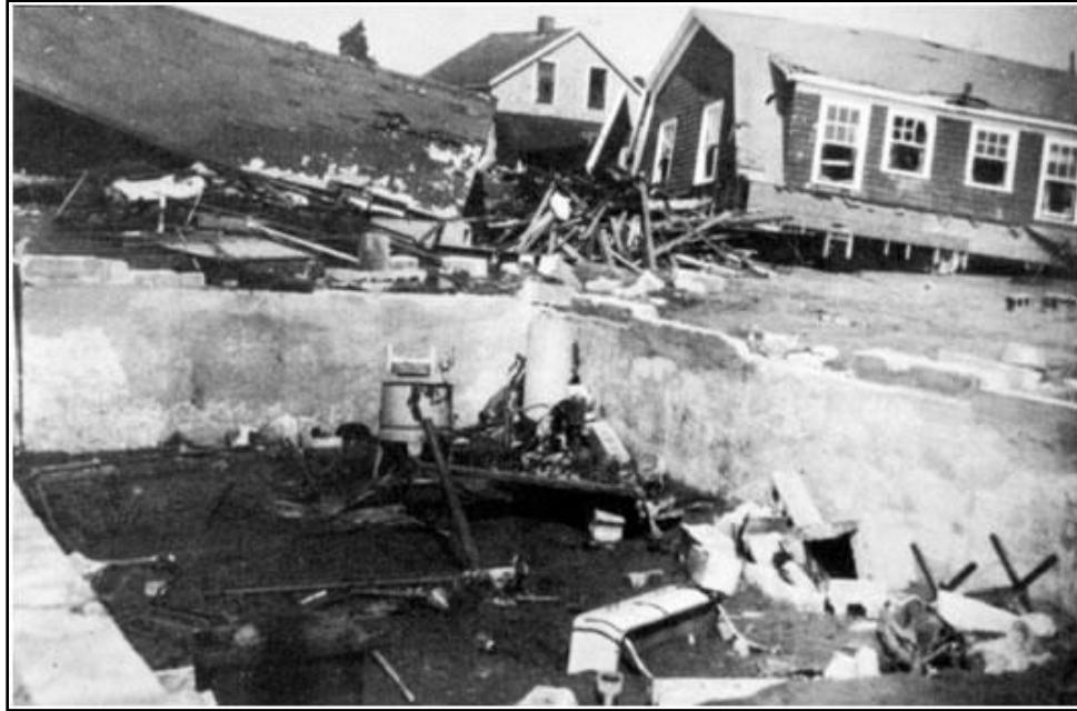
Figure 1-7: The remains of houses in Island Park, Rhode Island after the hurricane of 1938. (Source NOAA)
