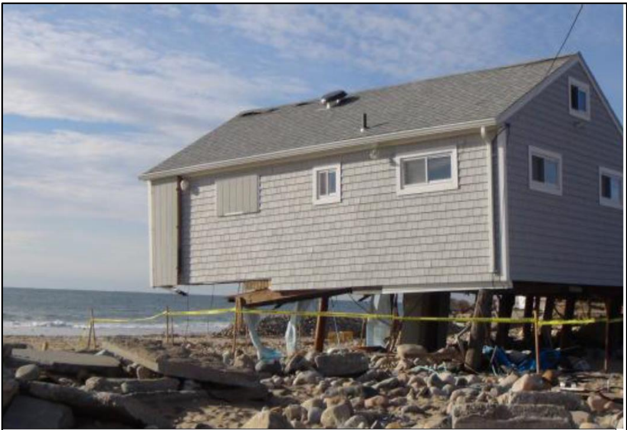
Figure 1-9: Damaged home in Westerly, Rhode Island after Superstorm Sandy (October 2012).
