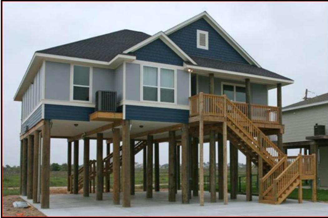
**Figure B 7-5:** Structure elevation example
