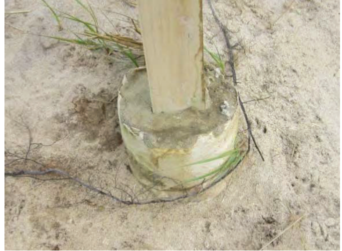
Close up of exposed concrete at base of sign.
