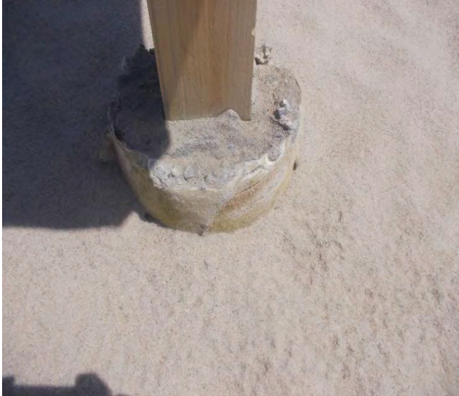
Minor erosion at base. Relatively slight deterioration relative to June 2017.
