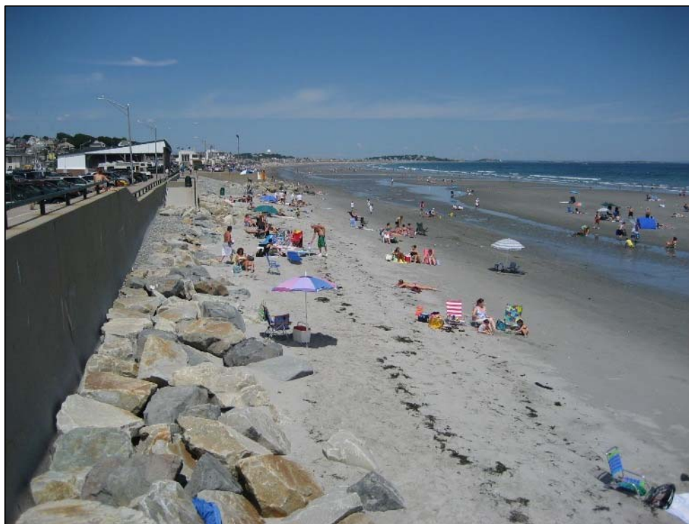
Figure 7-18. Beach in southern section of the seawall with existing toe protection during low tide (July 2007).
