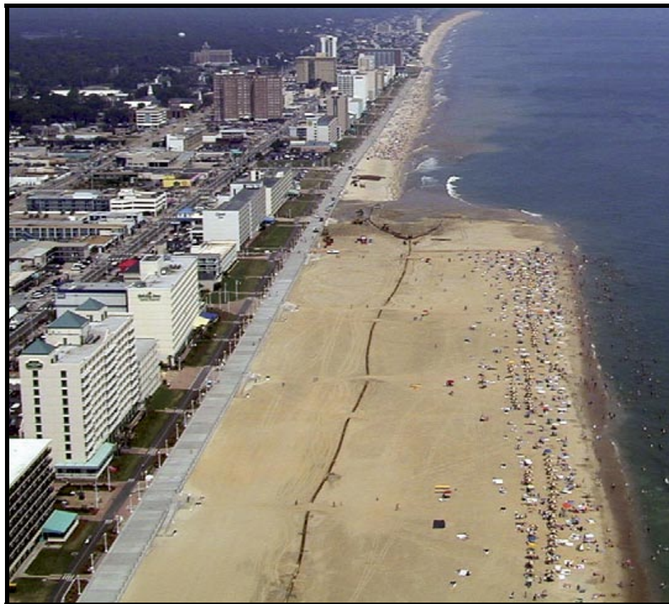
Figure 6-2. Beach nourishment project under construction in Virginia Beach, VA (photo courtesy of Virginia Beach).
