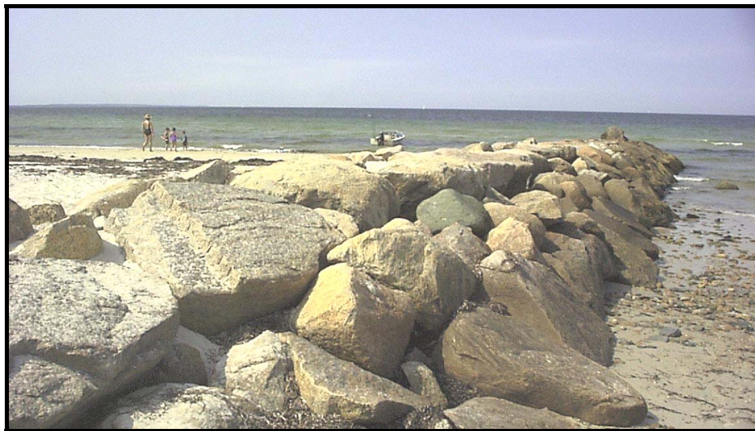
Figure 6-8. Existing groin showing updrift accretion fillet (left side of groin) and downdrift erosion zone (right side of groin). These shoreline conditions are typical in areas of groins.
