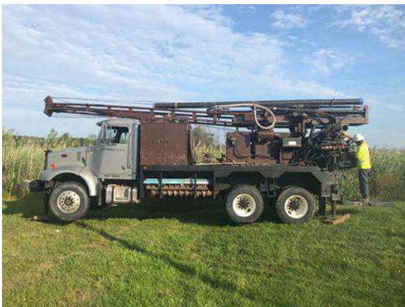
Rig setting up to install MW9BR
