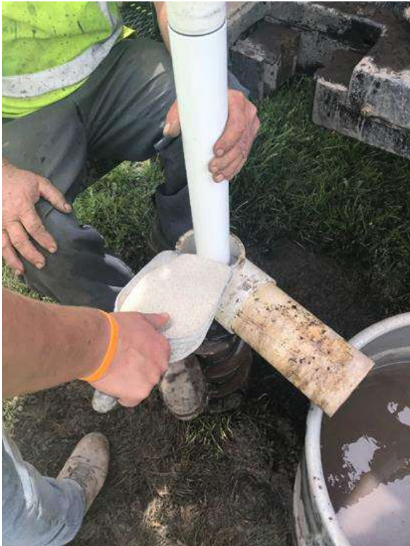
Filter pack sand being placed around the screen.
