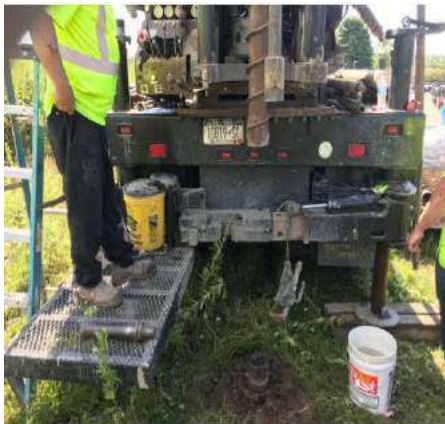
Drill rig setting up to perform split-spoon sampling at MW16.
