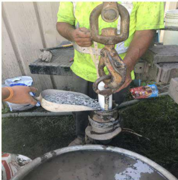
Bentonite pellet seal being placed above the filter pack sand.
