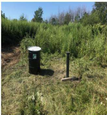
Well completion at MW16 with protective stickup casing. Labeled nonhazardous drum containing soil cuttings.
