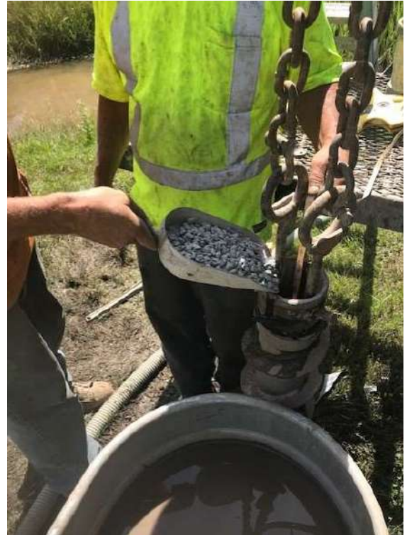
Bentonite pellet seal being placed above the filter pack sand.
