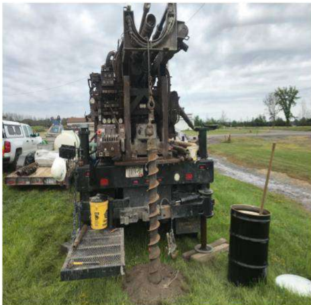
Auger set up at MW 6
