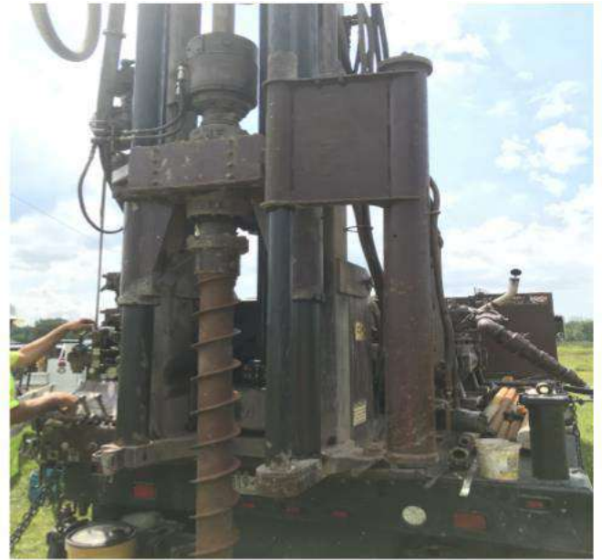
Auguring to below ground surface at MW10
