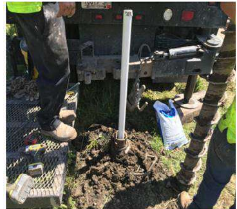
PVC screen/riser installation at MW16.
