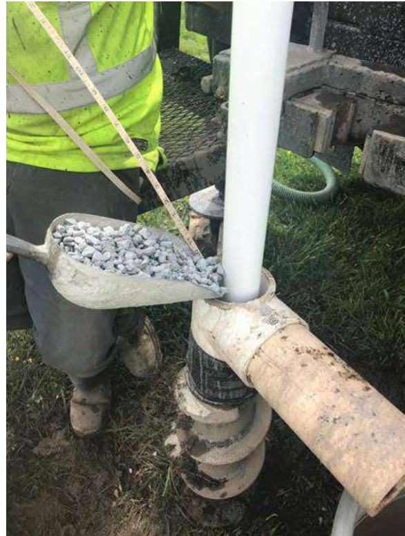
Bentonite pellet seal being placed above the filter pack sand.
