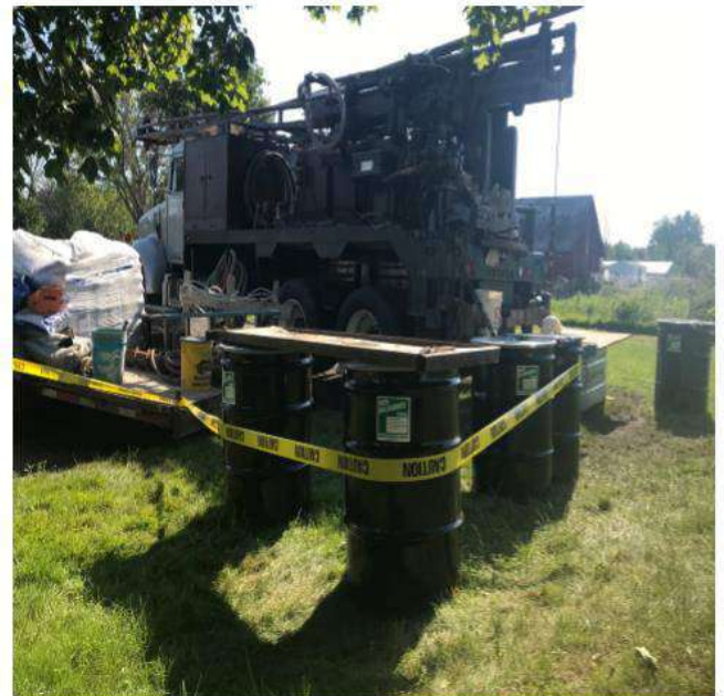
MW5BR drilling site with restricted access. Includes labeled non-hazardous investigation derived waste drums for soil cuttings and groundwater.
