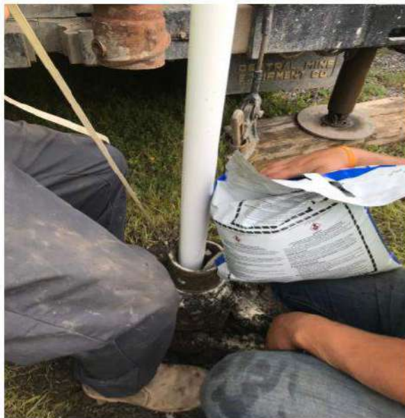
Filter pack installation (#00 silica) at MW13
