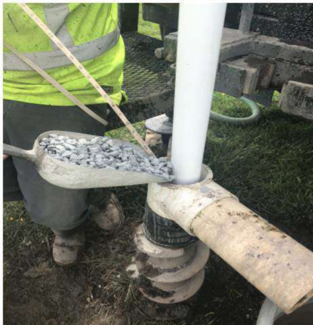
Adding bentonite chips to MW5BR
