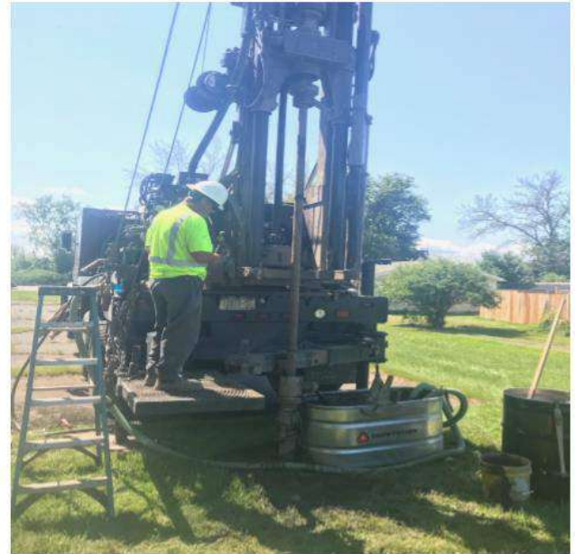
Rock coring at MW5BR
