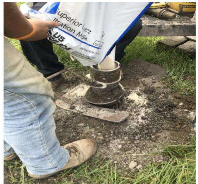
Bentonite seal application at MW10
