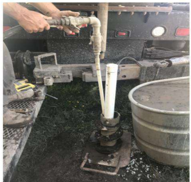
Borehole grouting above bentonite pellet seal using a tremie pipe.
