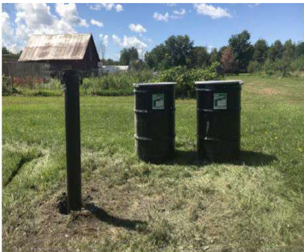
Well completion at MW5OB with protective stick-up casing. Includes labeled non-hazardous investigation derived waste drums for soil cuttings.
