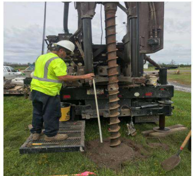
Augering below ground surface at MW 6.
