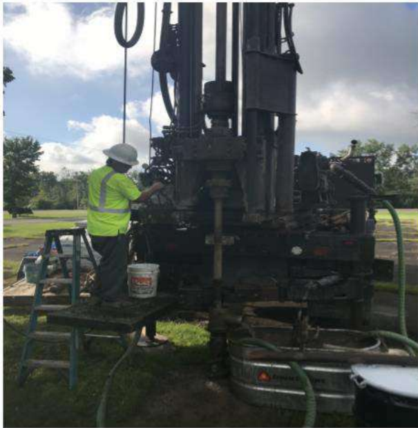
Additional rock coring at MW5BR (34-39' bgs)
