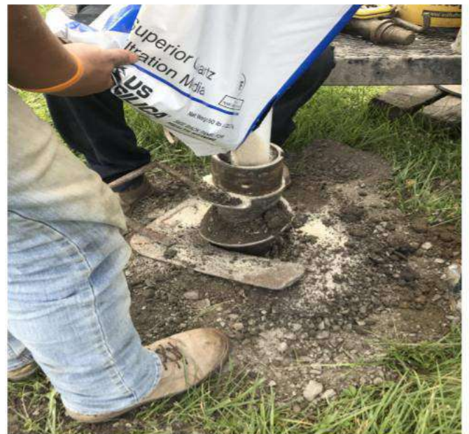
Bentonite seal application at MW10
