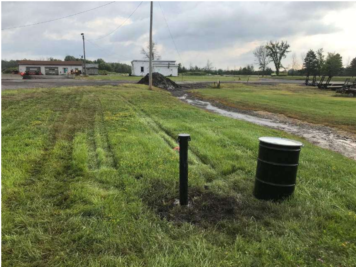
Well completion at MW6 with protective stick-up casing and one drum of non-haz soil cuttings.
