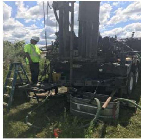
Rock coring at MW1BR
