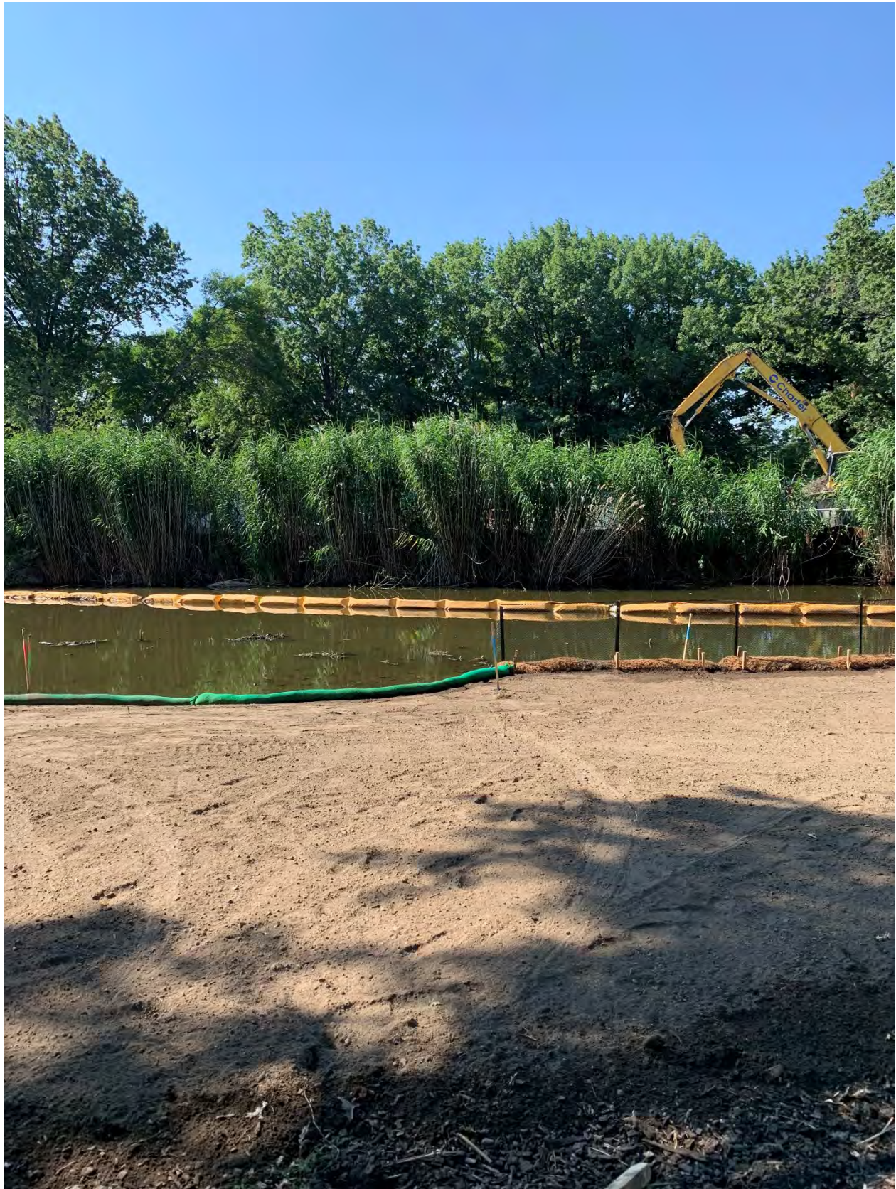
Work Area #11 – section of river immediately downstream of Work Area #10 – herbivore fence, coir log, and loam installed ready for seeding and plant installation. Note the phragmites on the opposite bank which will be removed now as part of additional work added to the project, starting in October 2022.
