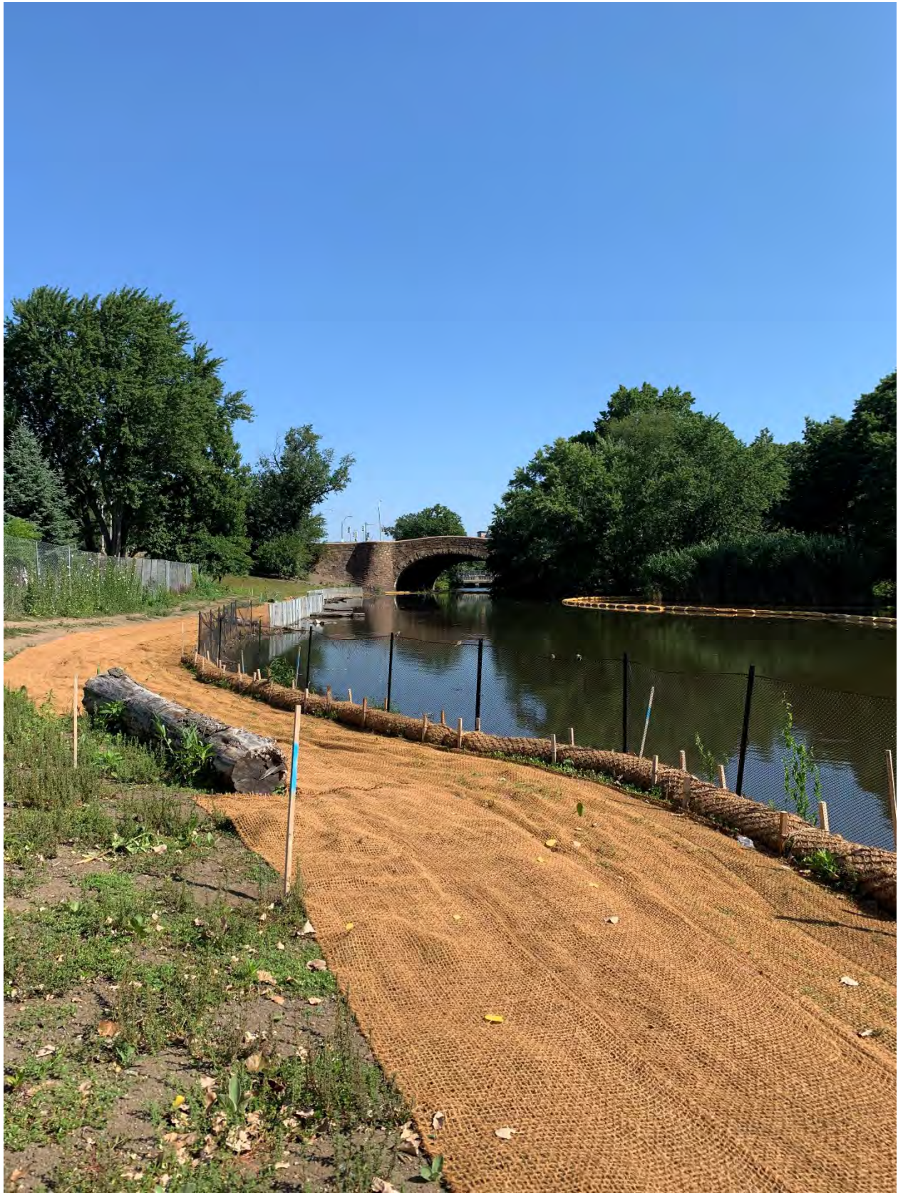
Work Area #12 – section of river upstream of Boylston Street Bridge – herbivore fence, coir log, turf reinforcement mattress (TRM), habitat log, and loam installed ready for seeding and plant installation.
