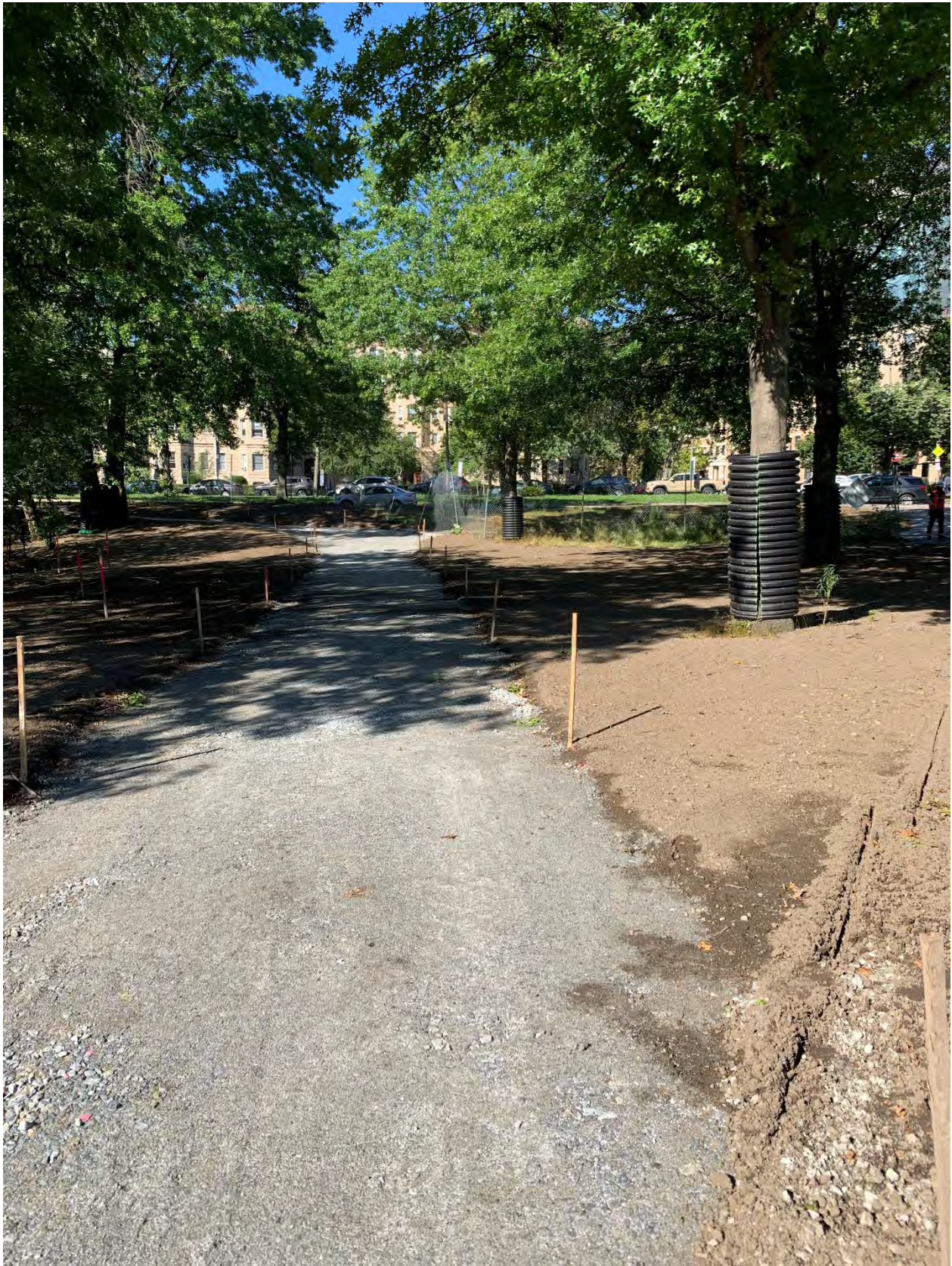
Work Area #11 – section of river immediately downstream of Work Area #10 – reconstructed stonedust pathway by the Victory Gardens. Note also the placed loam which is ready for seeding.
