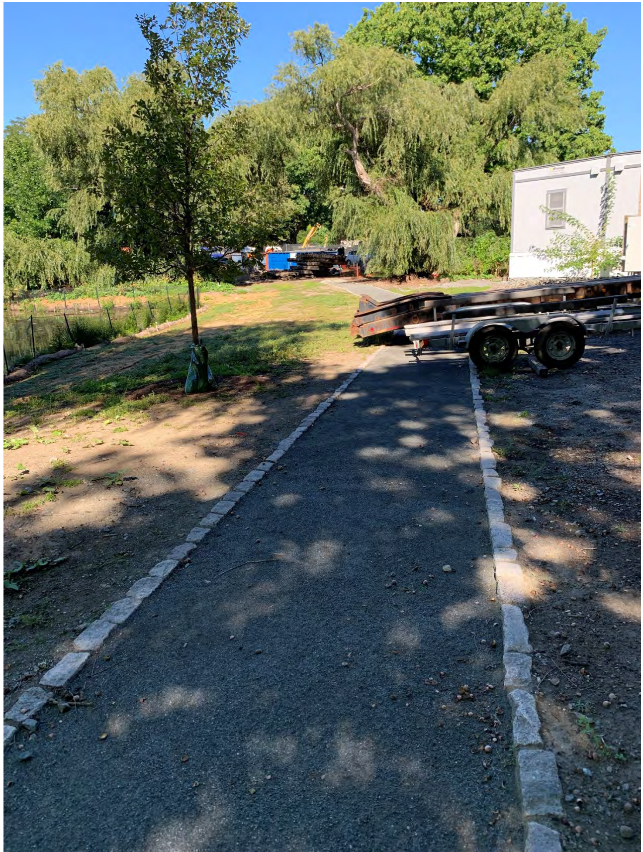
Work Area #10 – section of river immediately downstream of Work Area #9 which ends at Agassiz Road – reconstructed stonedust pathway behind the construction trailers. Note also the plantings and the bank which will need reseeding as part of the two-year guarantee period.
