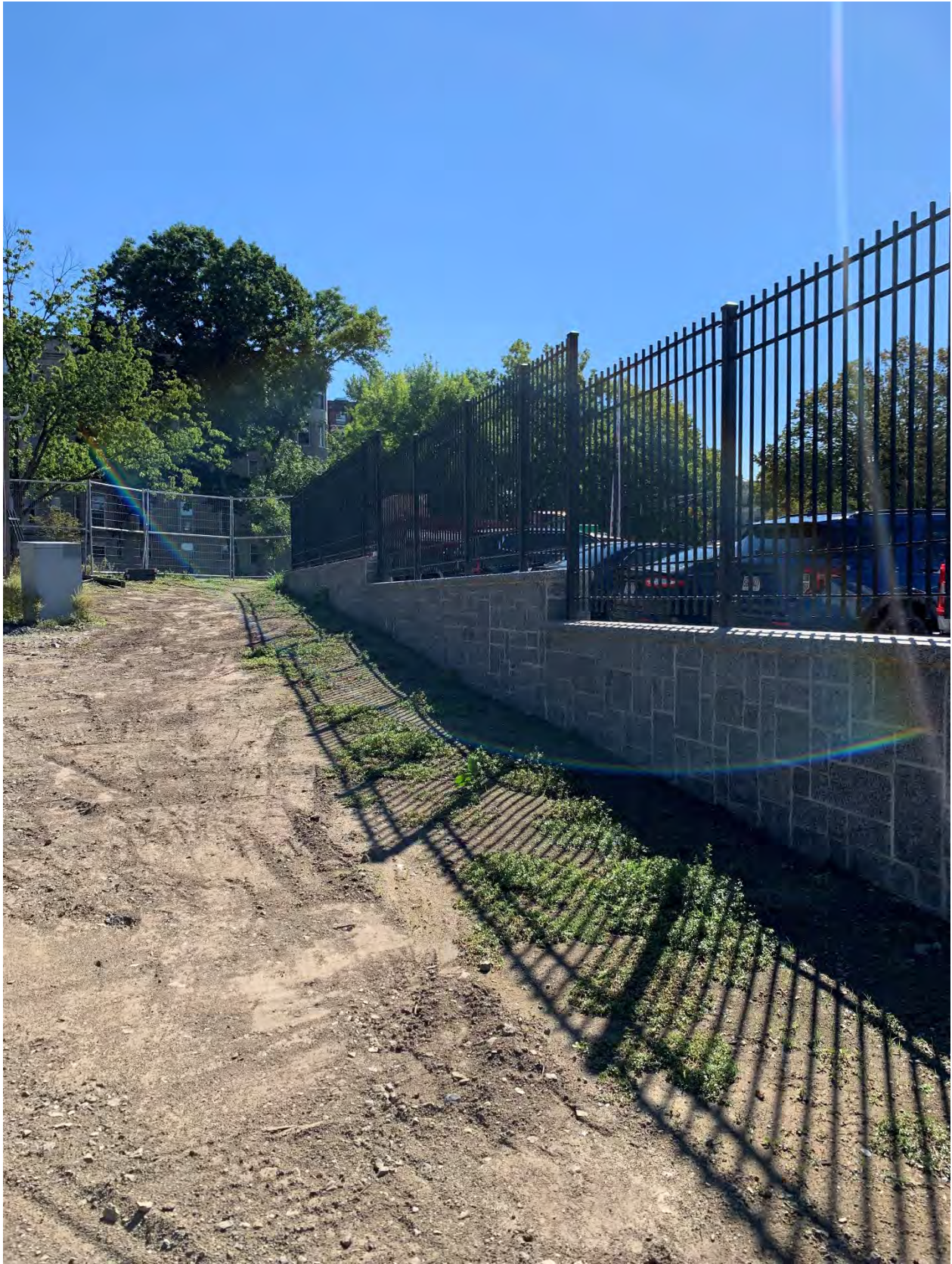
Work Area #13 – Boston Fire Department Building in the vicinity of the Fenway and Agassiz Road – security fence and granite veneer installed on the constructed floodwall.
