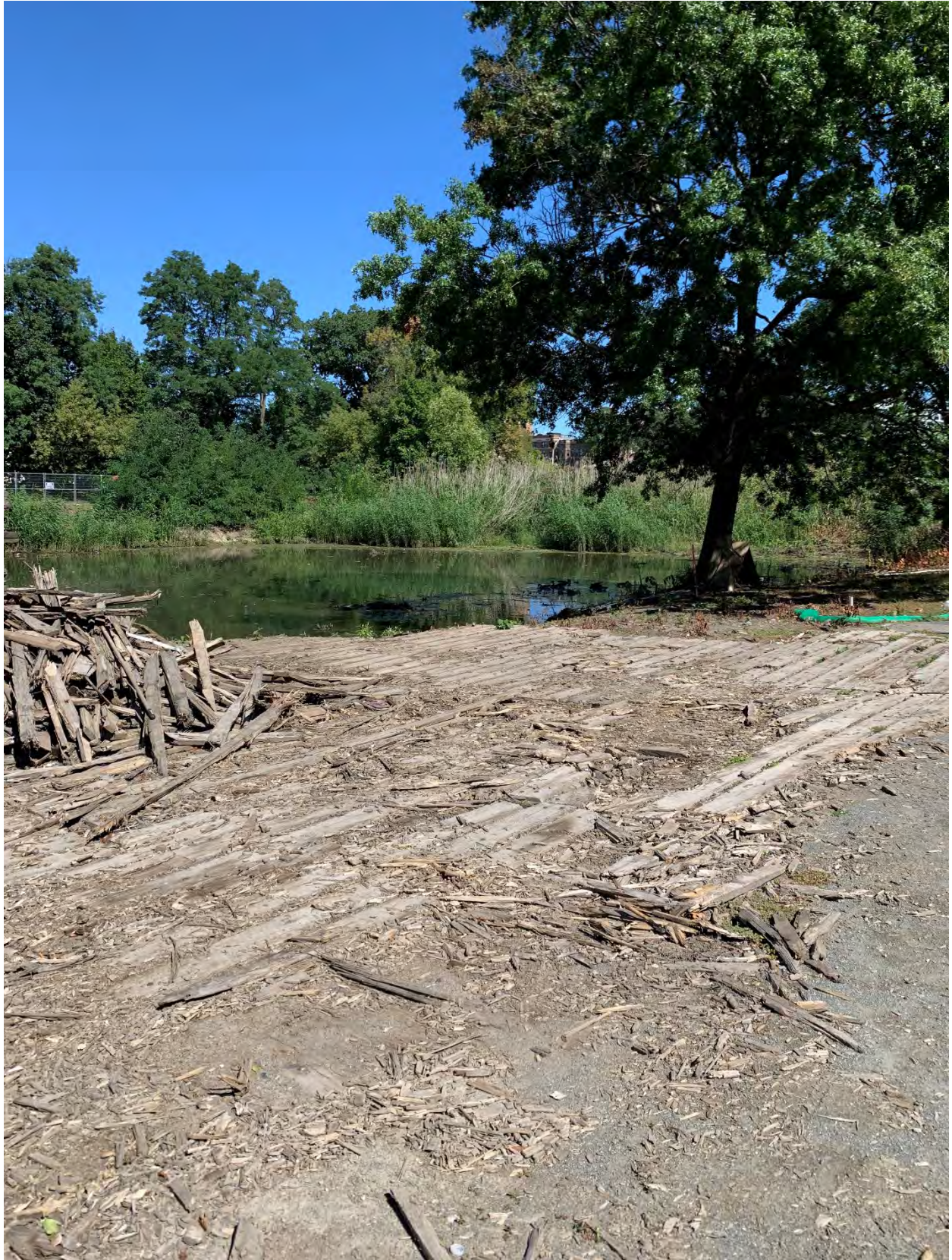
Work Area #6 – section of river by Back Bay Yard near the intersection of Park Drive and Riverway – flood risk management channel dredged up to the MWRA easement. Note the phragmites that is encroaching into the river that still needs to be removed in 2023.
