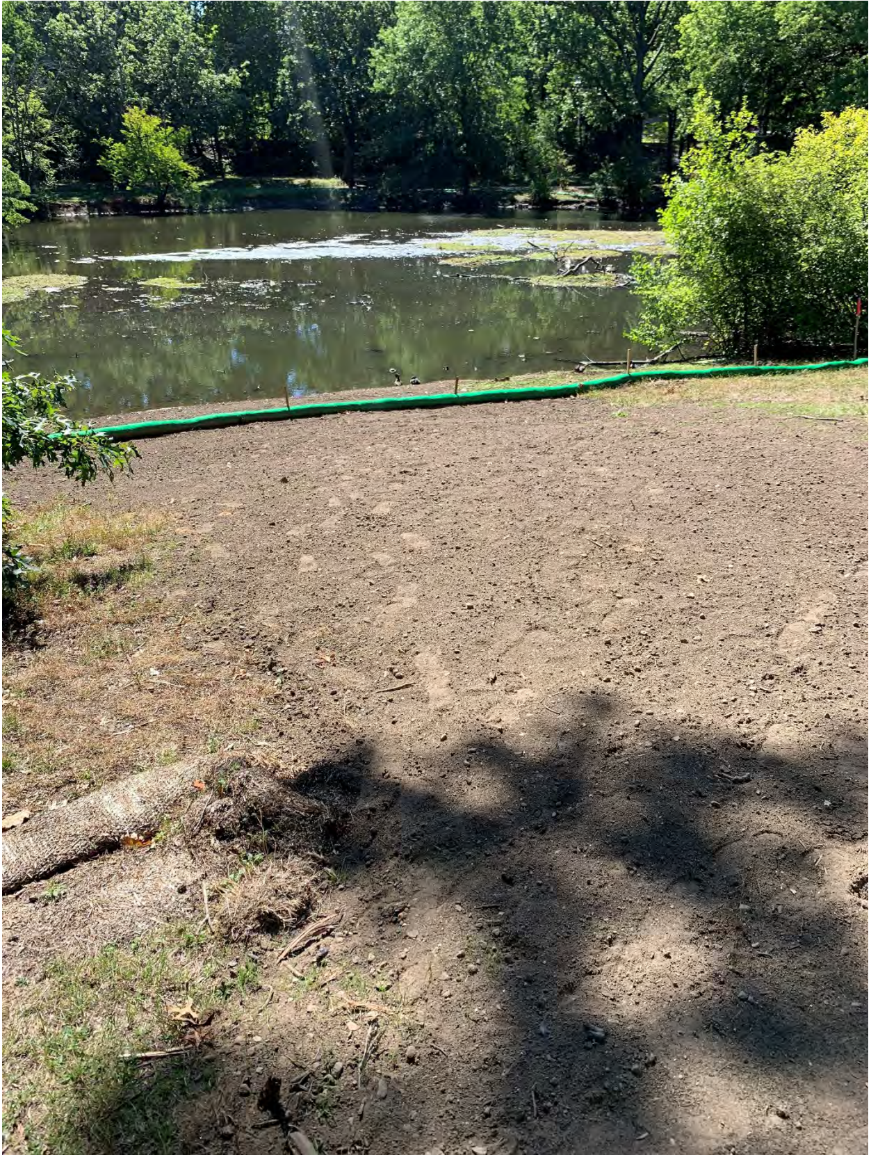
Work Area #5 – section of river by Short Street Bridge – phragmites removed as part of the additional work request by the Sponsors. This removal will provide additional environmental restoration benefits to the system as well as provide maintenance benefits for the dredged channel. Area loamed and ready for seeding.
