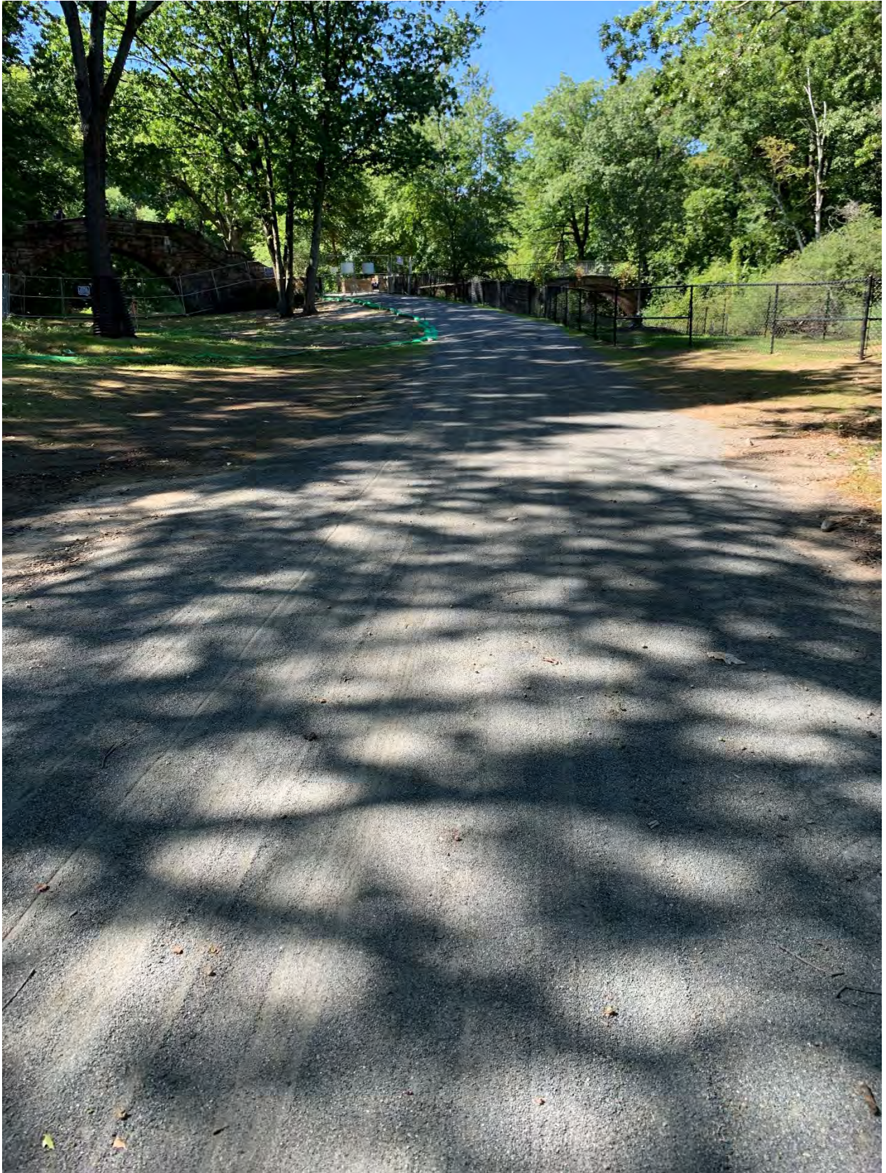
Work Area #5 – section of river by Short Street Bridge – reconstructed stonedust pathway.
