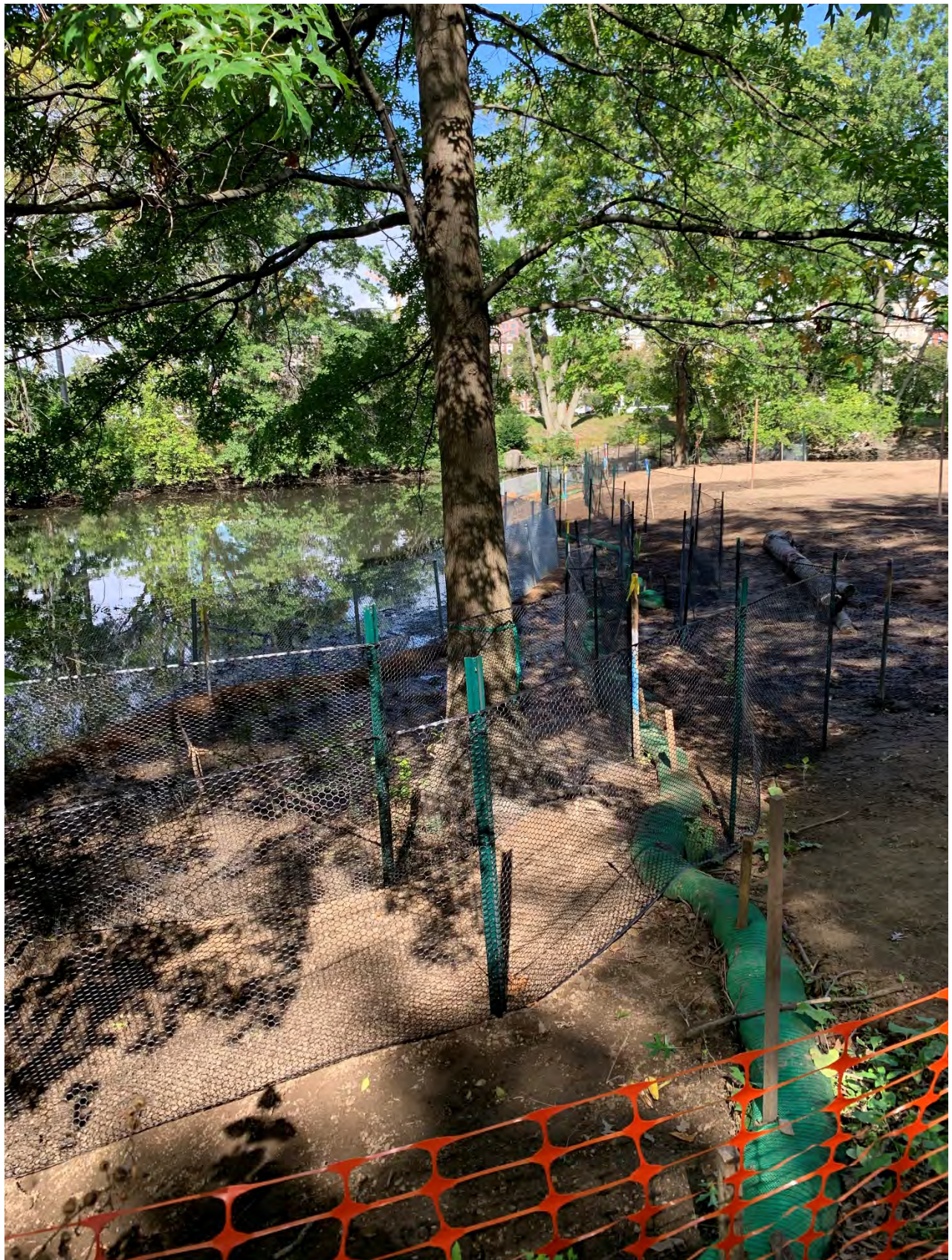
Work Area #9 – section of river immediately downstream of Work Area #8 – constructed wetland shelves A (pickerel weed emergent plants) and B (wetland seed mix). Note the layers of temporary herbivore deterrent fence and temporary in-channel carp deterrent fence to allow for plant establishing during the two-year guarantee period.
