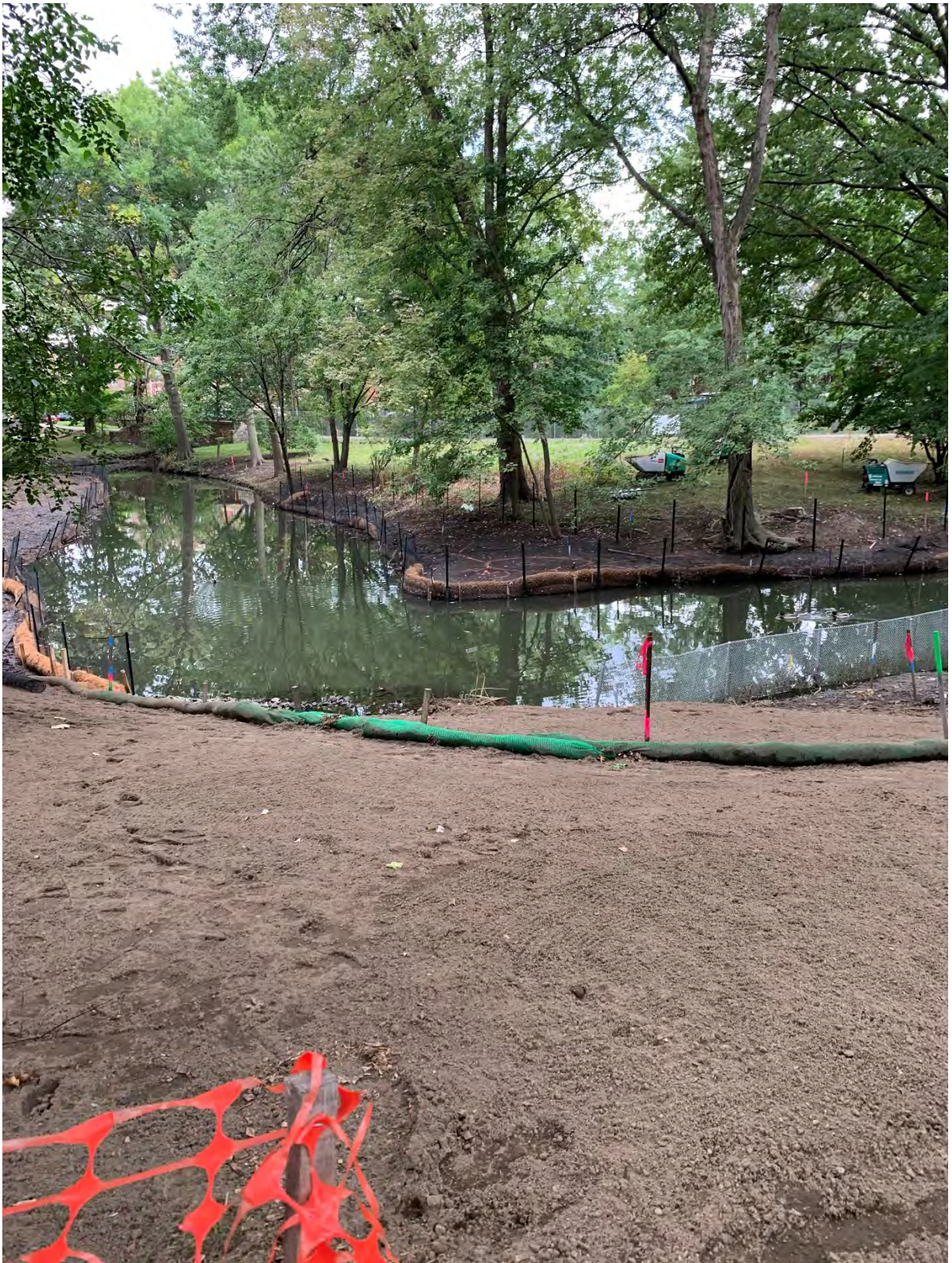
Work Area #3 – section of river at Brookline Avenue, the Riverway, and Netherlands Road – near Beth Israel Deaconess Hospital – view of graded bank on the near side and across the river is the constructed wetland shelf with coir log. Also installed is the temporary herbivore deterrent fence.
