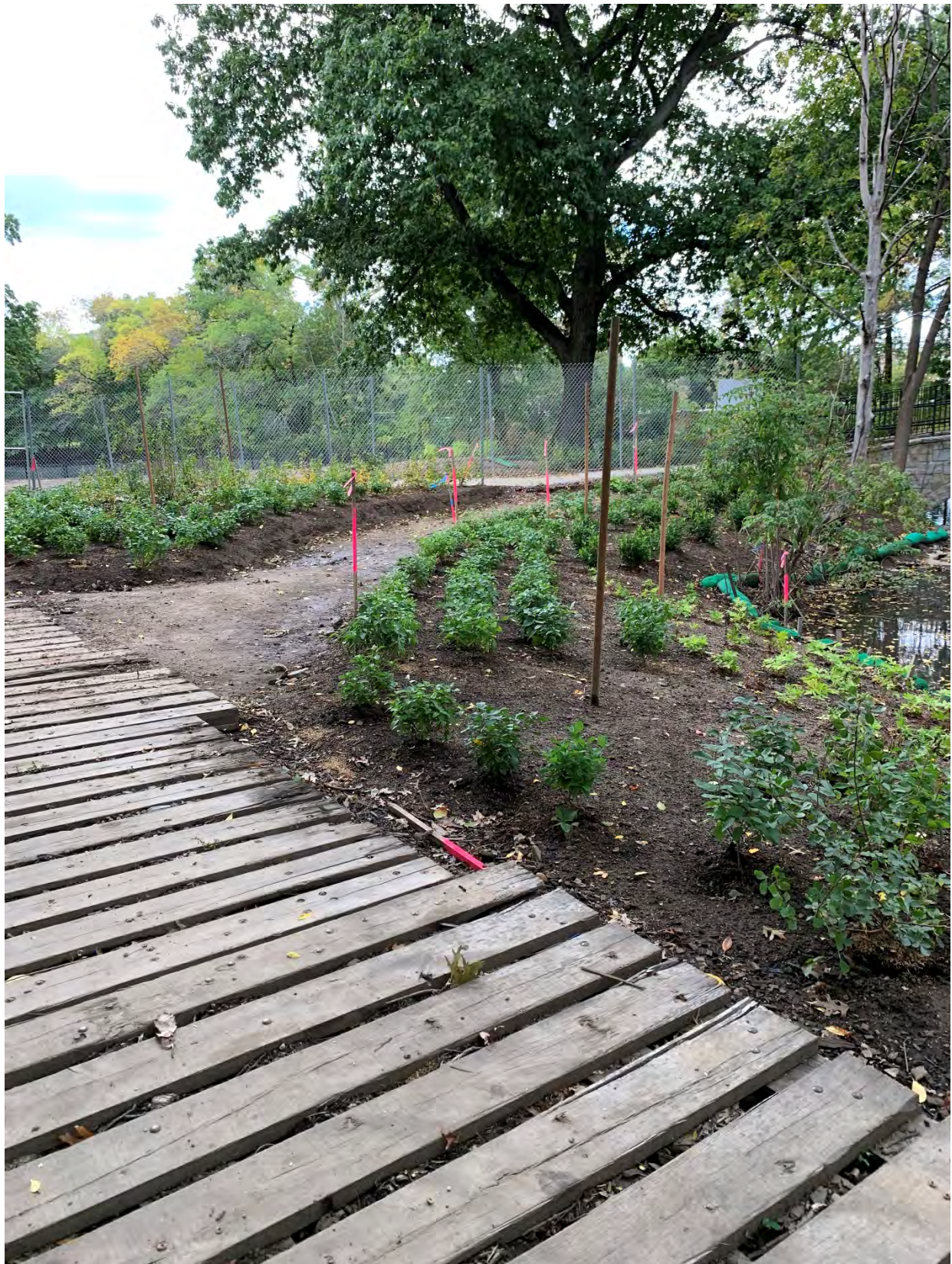
Work Area #9 – section of river immediately downstream of Work Area #8 – constructed shrub beds for restoration and the existing stonedust pathway which will also be restored. Note the long pole which designates the new tree location.
