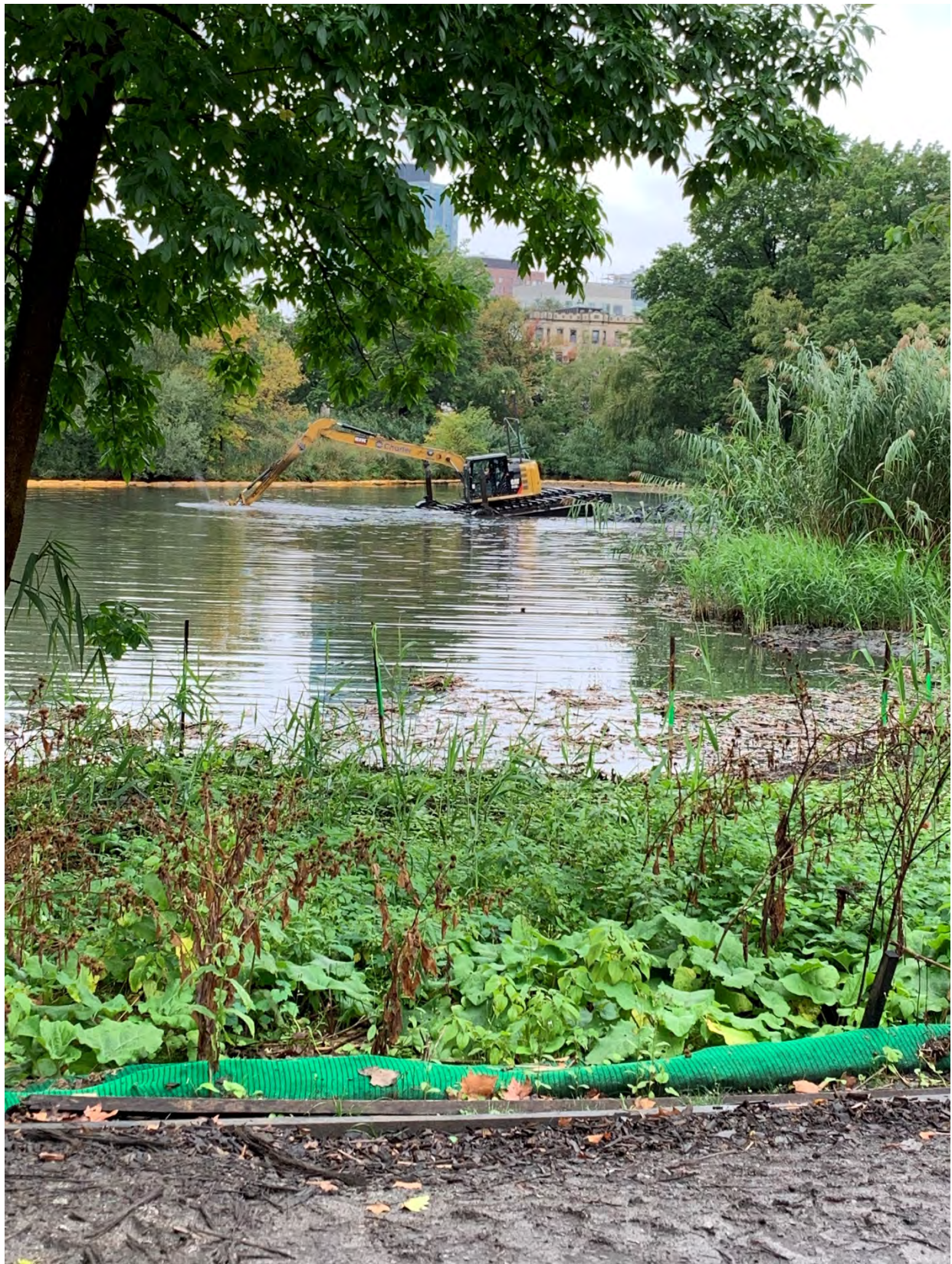
Work Area #10 – section of river immediately downstream of Work Area #9 which ends at Agassiz Road – amphibious excavator dredging the sediment from the river.
