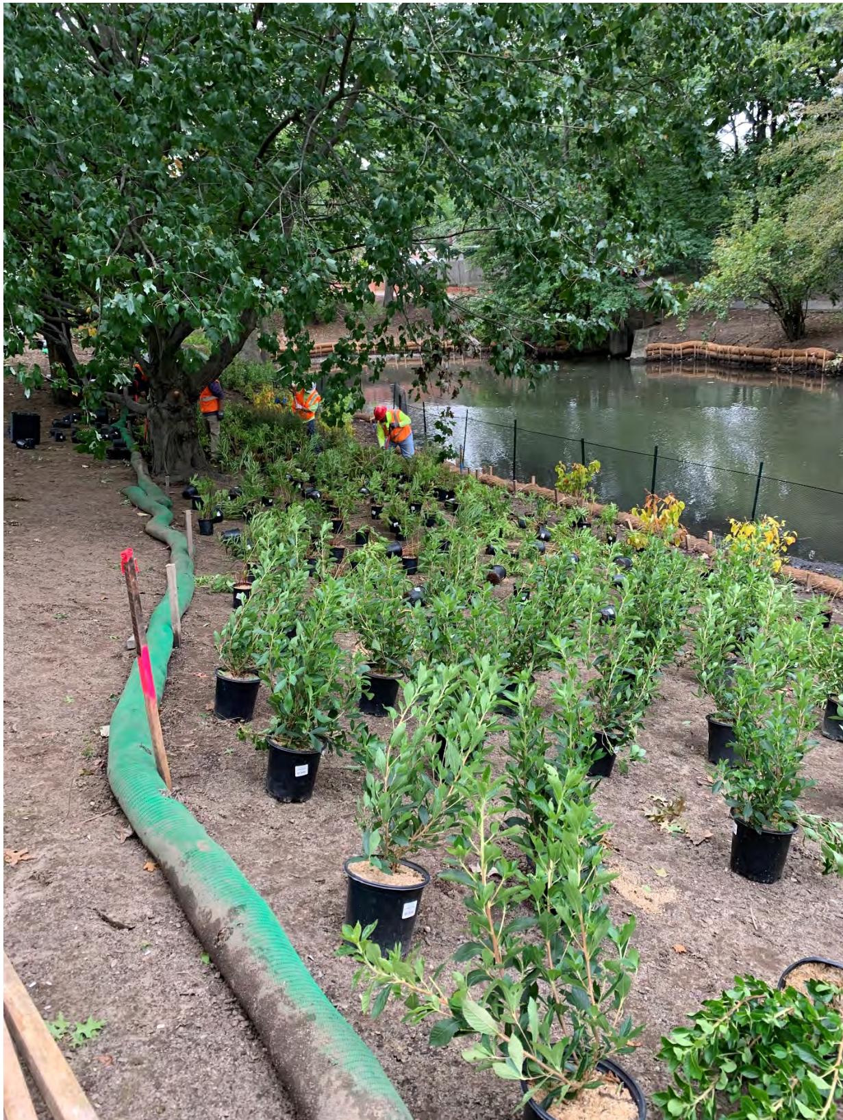
Work Area #4 – section of river immediately downstream of Work Area #3, across Netherlands Road – landscapers installing plants on the graded bank which are laid out by the landscape architect.
