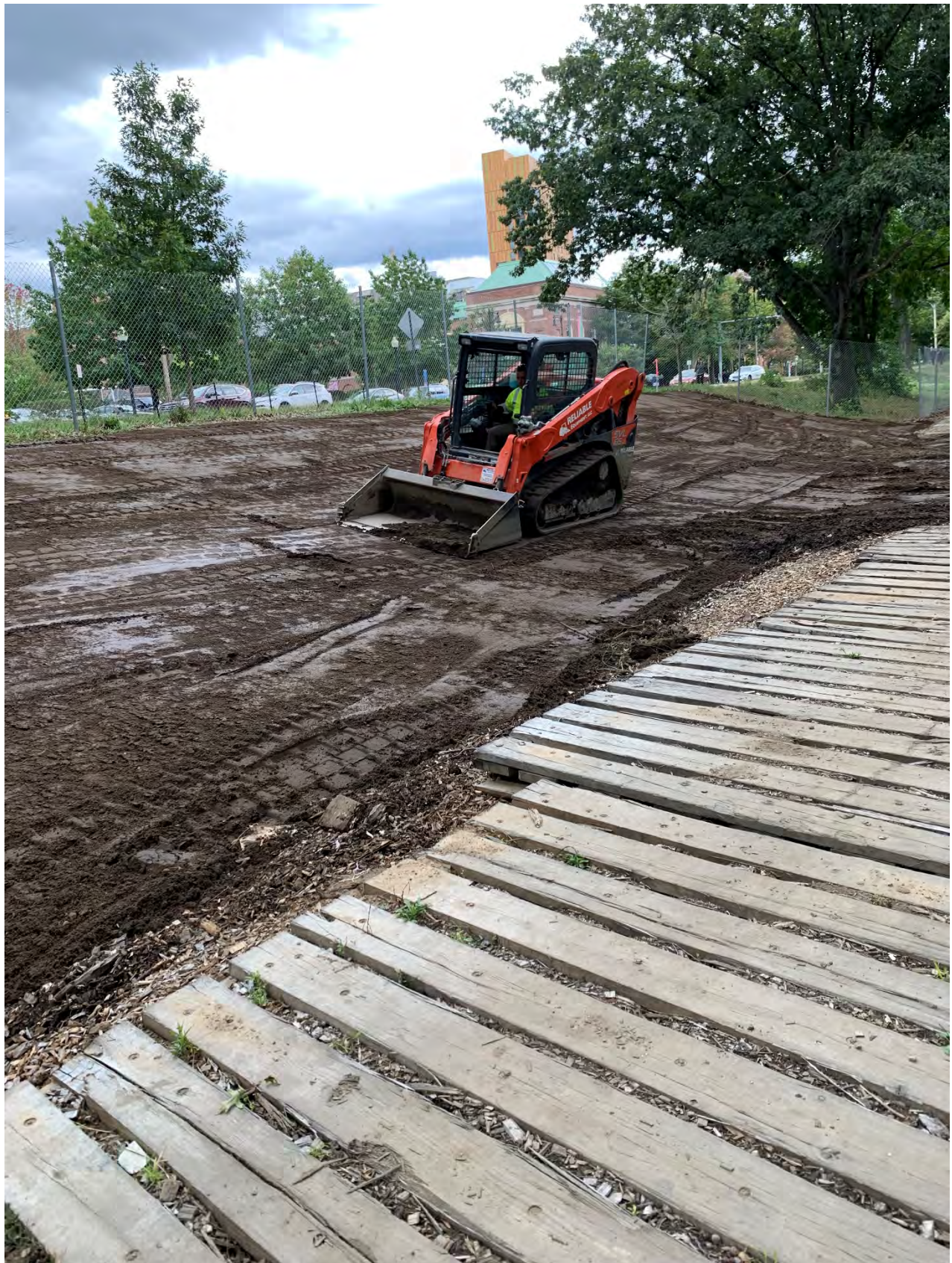
Work Area #8 – section of river downstream of Work Area #7 which is immediately downstream of Avenue Louis Pasteur – grading of the storage and staging area for restoration. Seed will be put down shortly.
