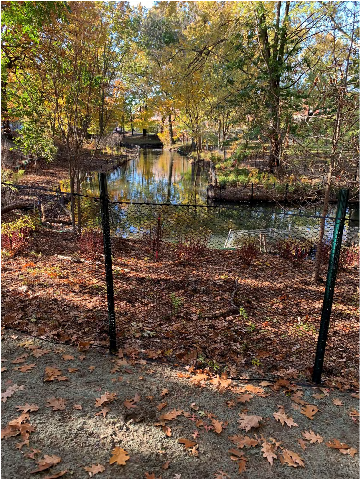
Work Area #3 – section of river at Brookline Avenue, the Riverway, and Netherlands Road – near Beth Israel Deaconess Hospital – view of planted bank on the near and far side and across the river is the constructed wetland shelf with coir log. Also installed is the temporary herbivore deterrent fence.
