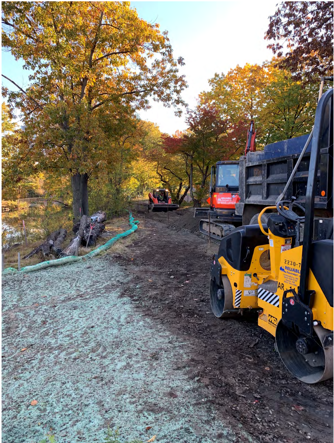
Work Area #9 – section of river immediately downstream of Work Area #8 – stonedust pathway restoration – grading and reconstruction of the existing stonedust pathway.
