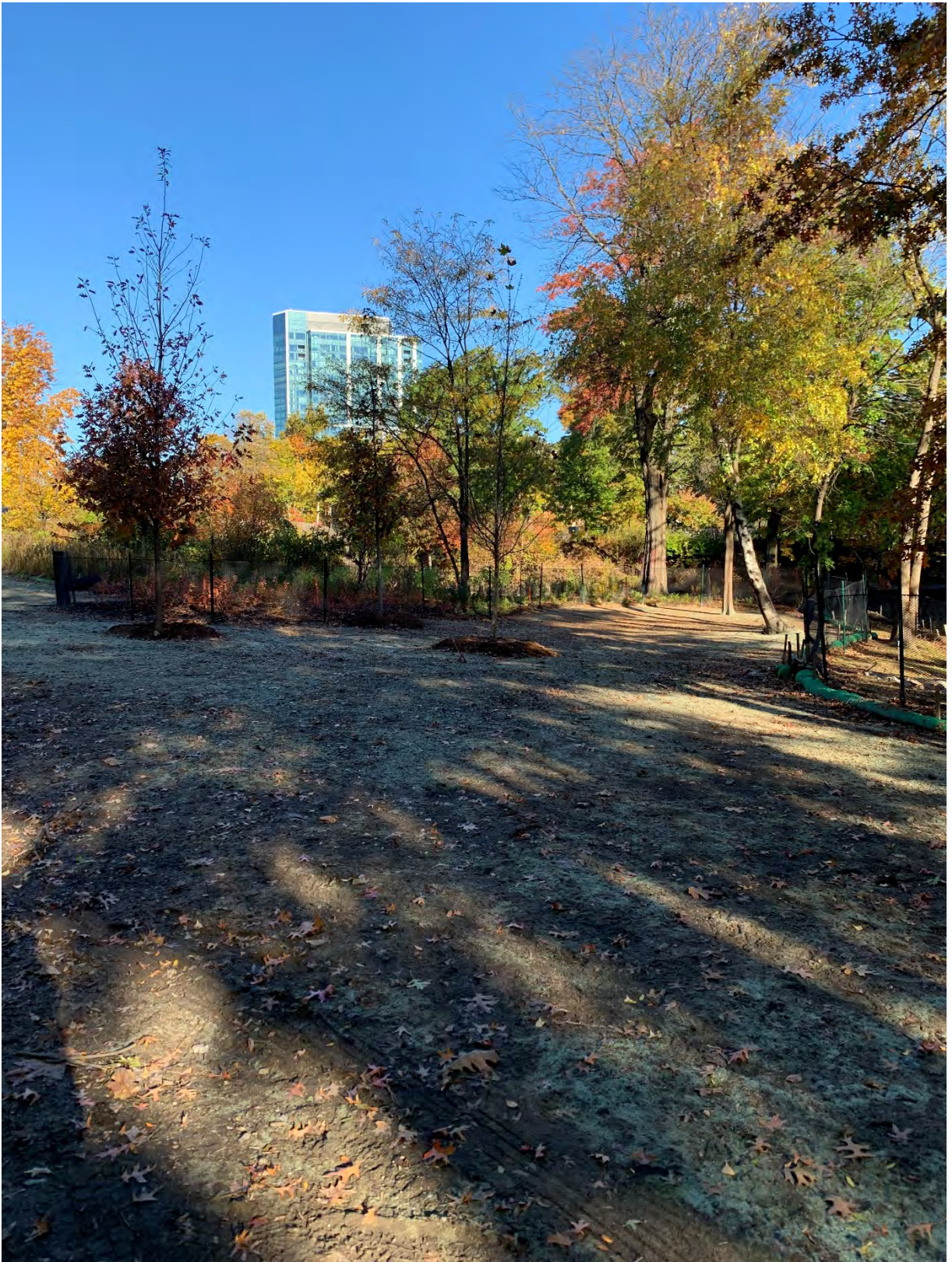
Work Area #7 – section of river immediately downstream of Avenue Louis Pasteur – newly planted trees and shrubs. Loam and hydroseed installed. Note also the herbivore deterrent fence to protect the planted shrubs during the two-year guarantee period.
