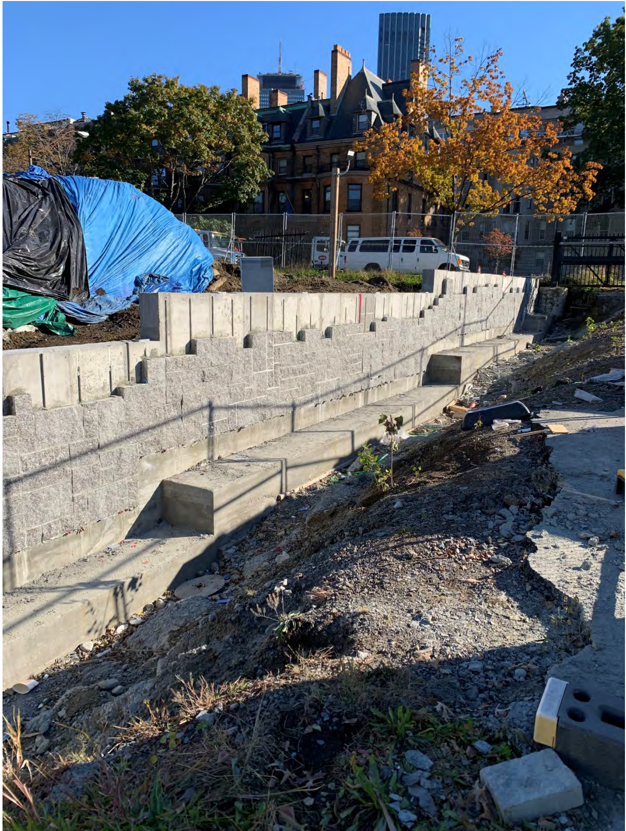
Work Area #13 – Boston Fire Department Building in the vicinity of the Fenway and Agassiz Road – granite veneer being installed on the newly constructed floodwall.
