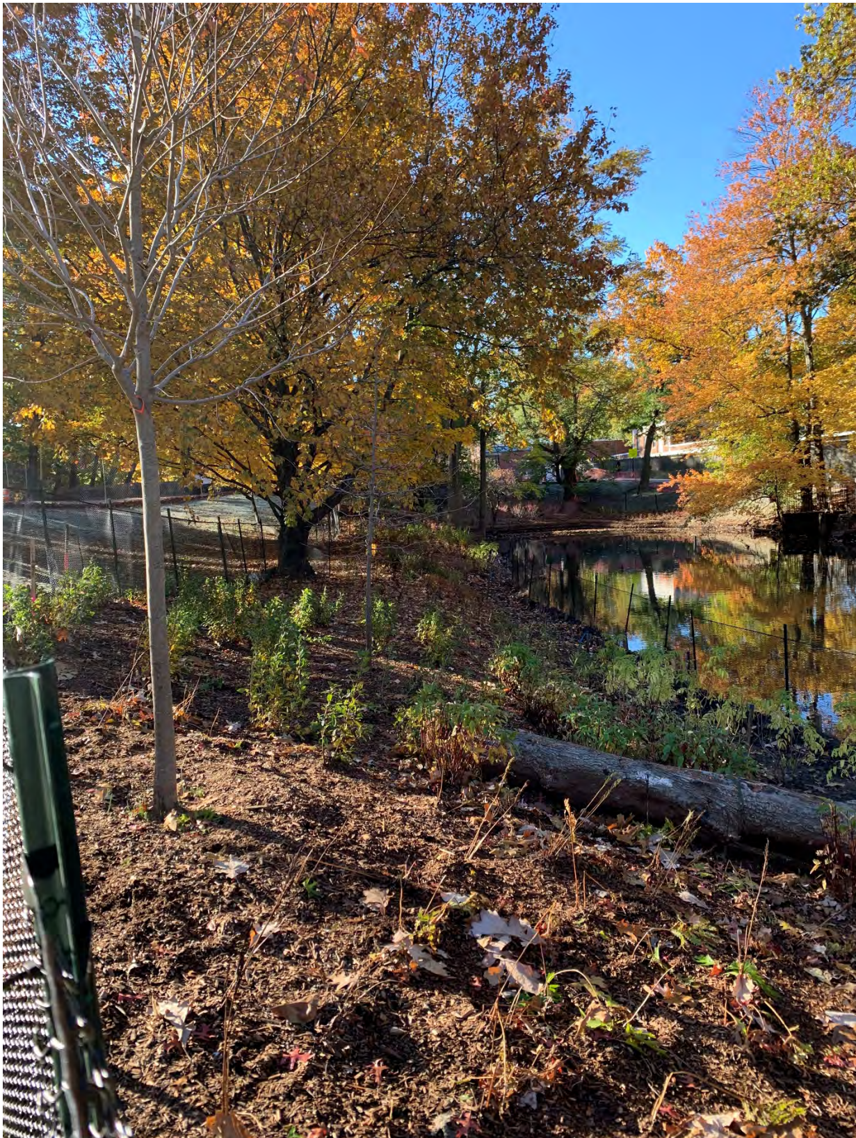
Work Area #4 – section of river immediately downstream of Work Area #3, across Netherlands Road – view of the planted bank with new tree and shrubs. Note also the habitat log on the bank as part of the restoration.
