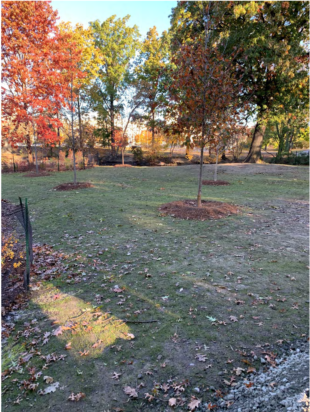
Work Area #9 – section of river immediately downstream of Work Area #8 – restored open area near pedestrian bridge. Note the newly planted trees and shrubs; and loam and seed in this area.
