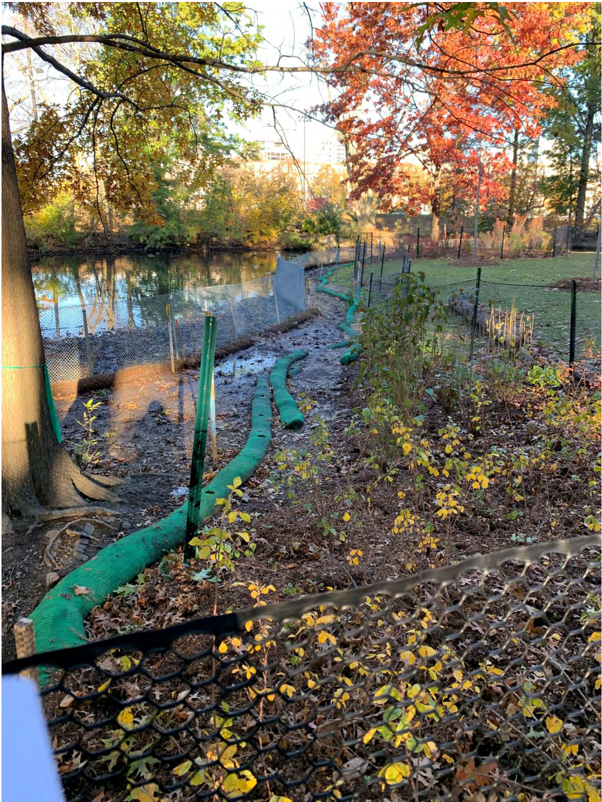
Work Area #9 – section of river immediately downstream of Work Area #8 – constructed wetland shelf A (pickerel weed emergent plants), wetland shelf B (wetland seed mix), and planted shrubs. Note the layers of temporary herbivore deterrent fence and temporary in-channel carp deterrent fence to allow for plant establishment during the two-year guarantee period.
