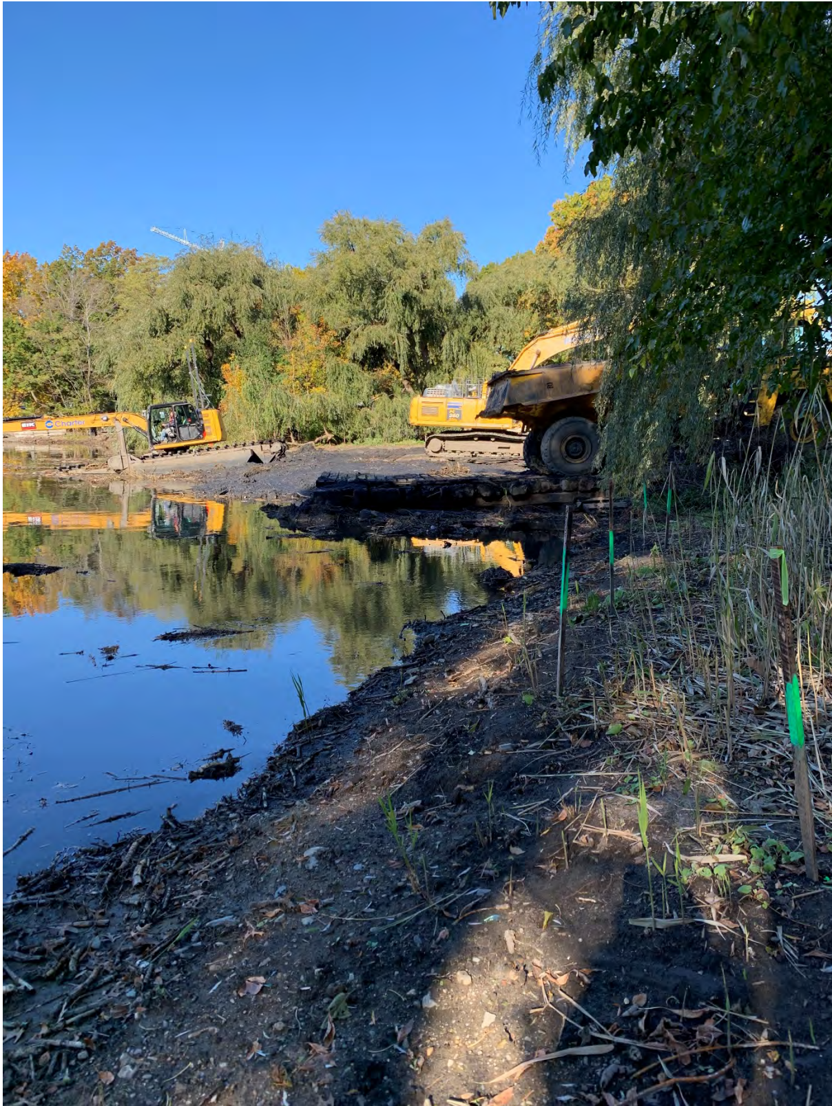
Work Area #10 – section of river immediately downstream of Work Area #9 which ends at Agassiz Road – sediment processing bins were removed as part of the dredging – steel sheeting removed and excavator will be dredging sediment in this location.
