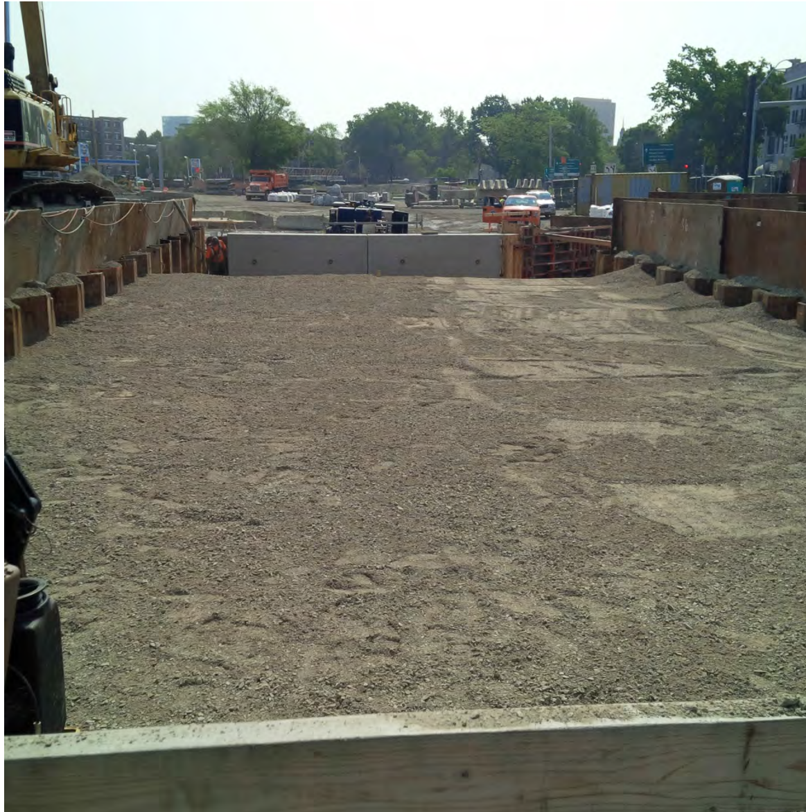
New Riverway precast concrete culvert is almost completely backfilled to grade. Note the backside of the downstream headwall – late August 2015.
