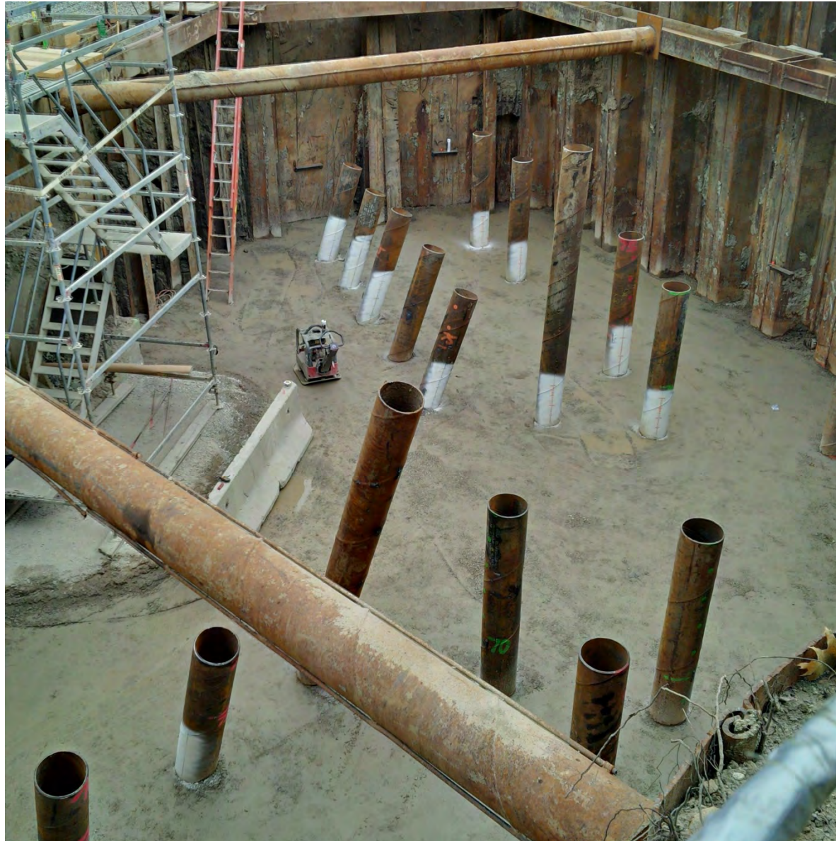
Installed pipe piles which will support the new upstream precast culvert sections that will be connected to the existing Avenue Louis Pasteur culvert – early September 2015.
