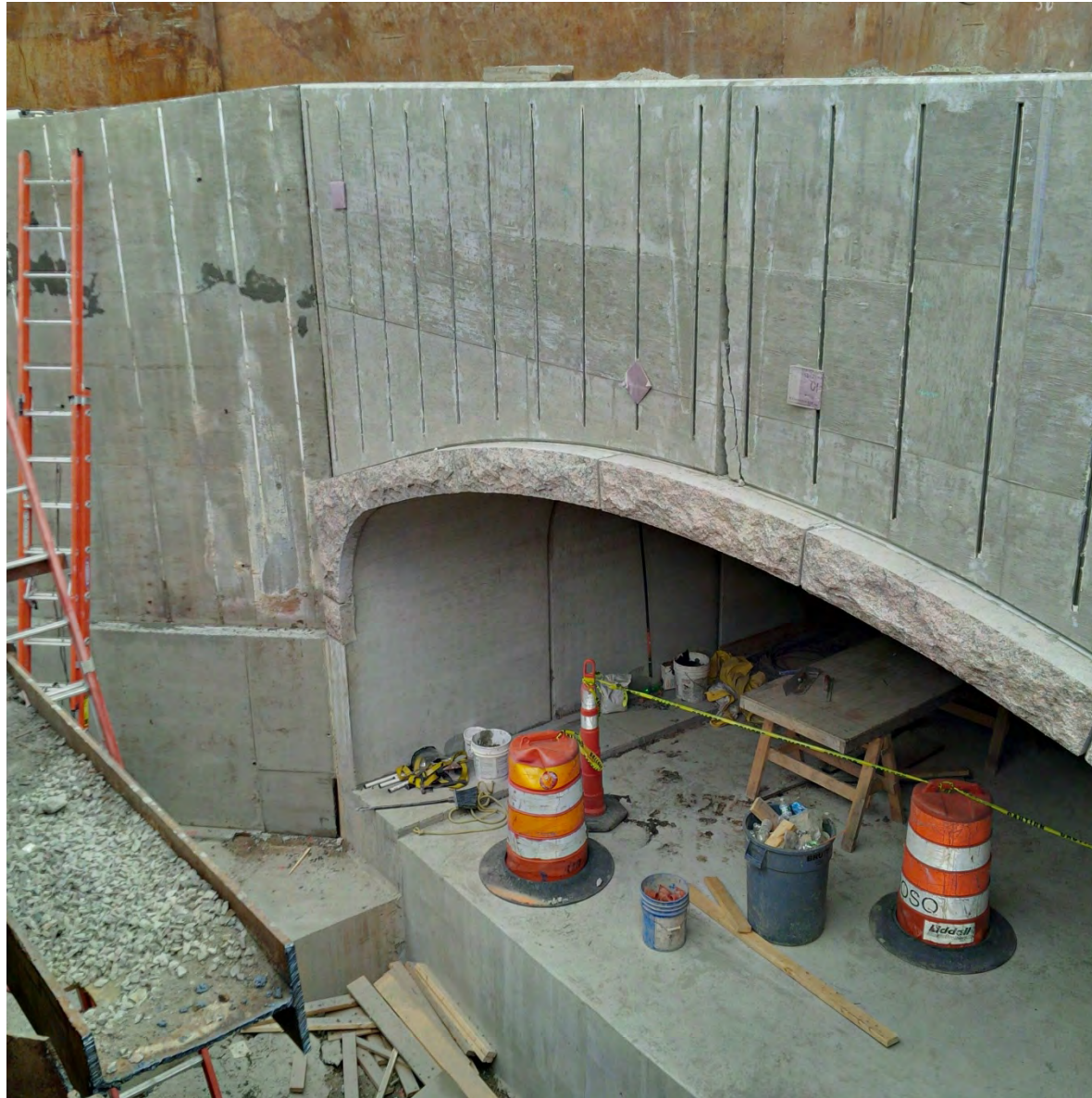
Downstream precast concrete headwall connected to the precast concrete Riverway culvert section. Note also the placed southeast concrete wingwall – late August 2015.
