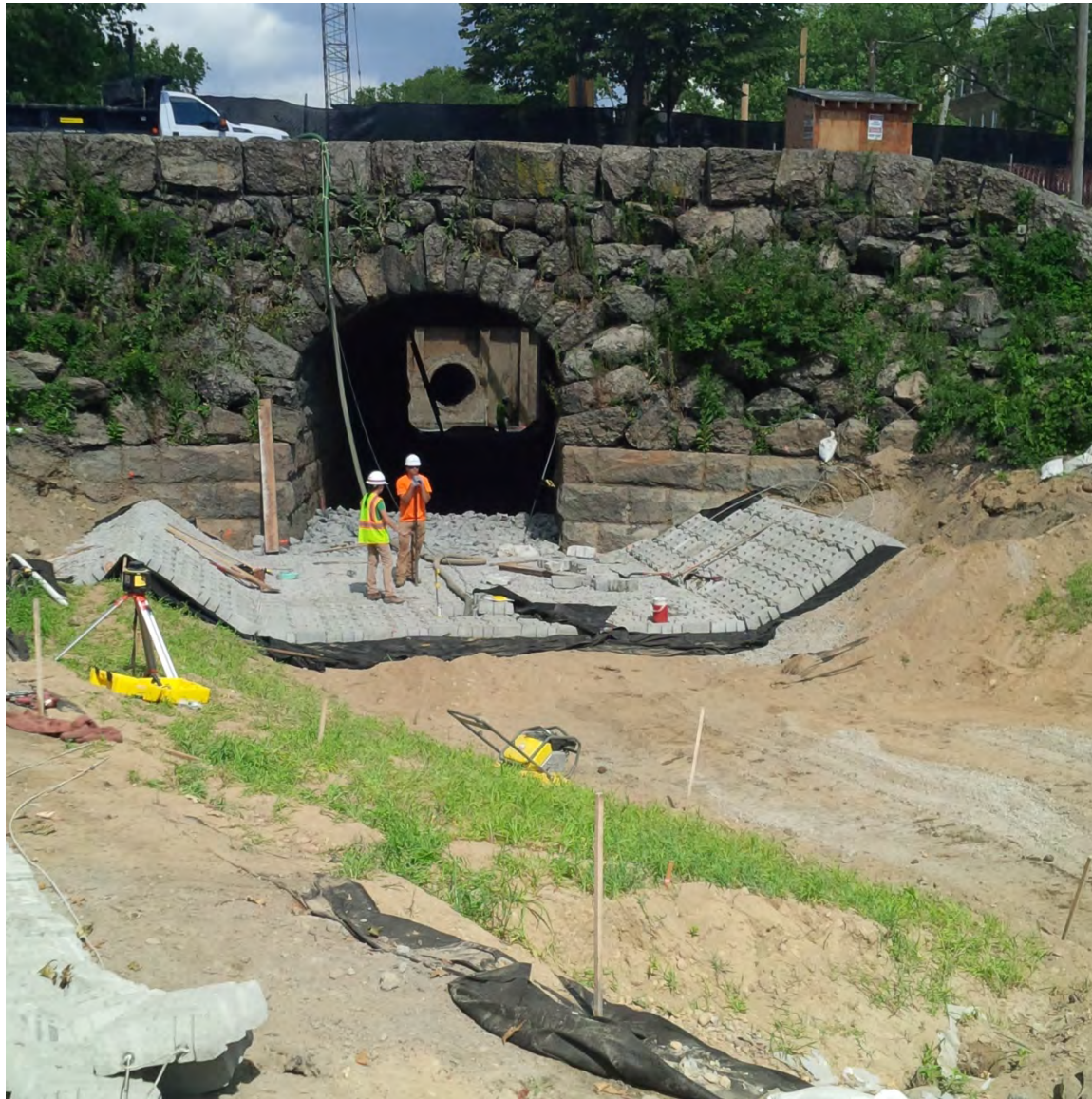
Downstream of Existing Avenue Louis Pasteur – sediment removed from inside the culvert; and installation of the articulated concrete blocks (ACB) has begun – late August 2015.
