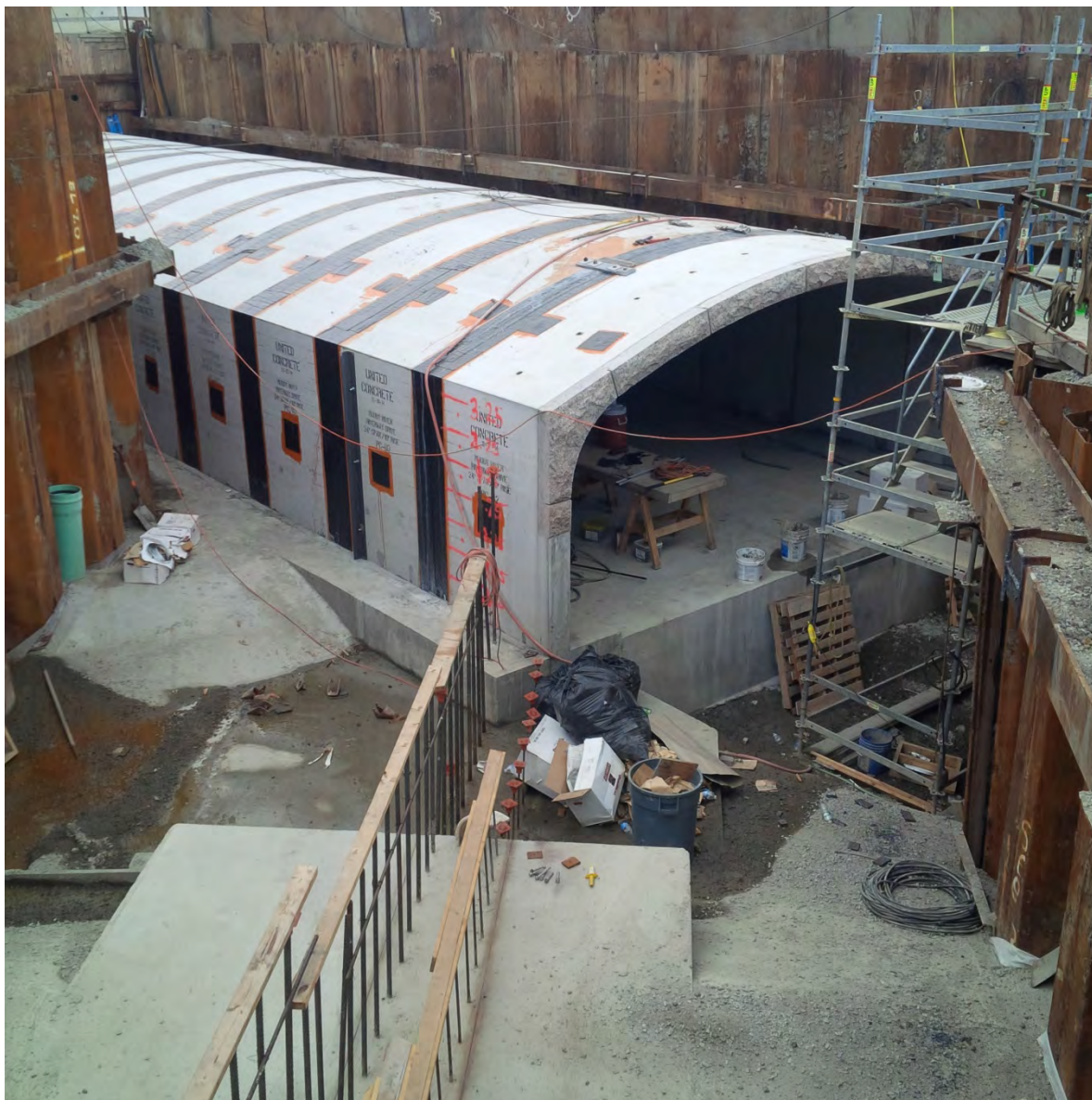
Waterproofing of the new precast concrete Riverway Culvert and rebar at the southeast wingwall – mid August 2015.
