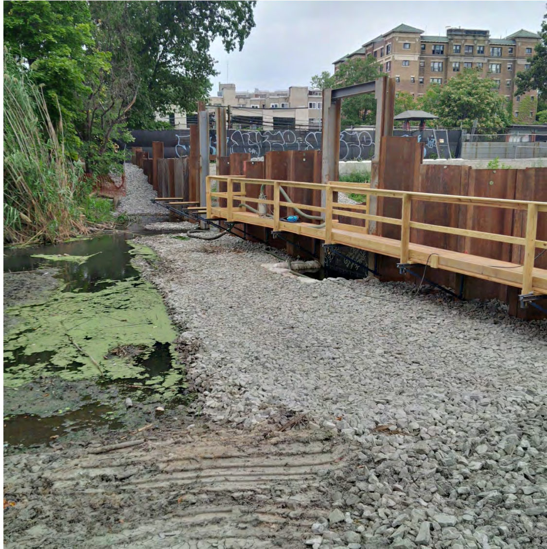
Upstream limits of Phase 1 Construction – line of steel sheeting installed as the Flow Restriction Control Structure (FRCS). Note the two weir opening in the sheeting to allow continuous flow over the structure; constructed walkway for maintenance of this structure; and scour protection of the FRCS with stone – early September 2015.
