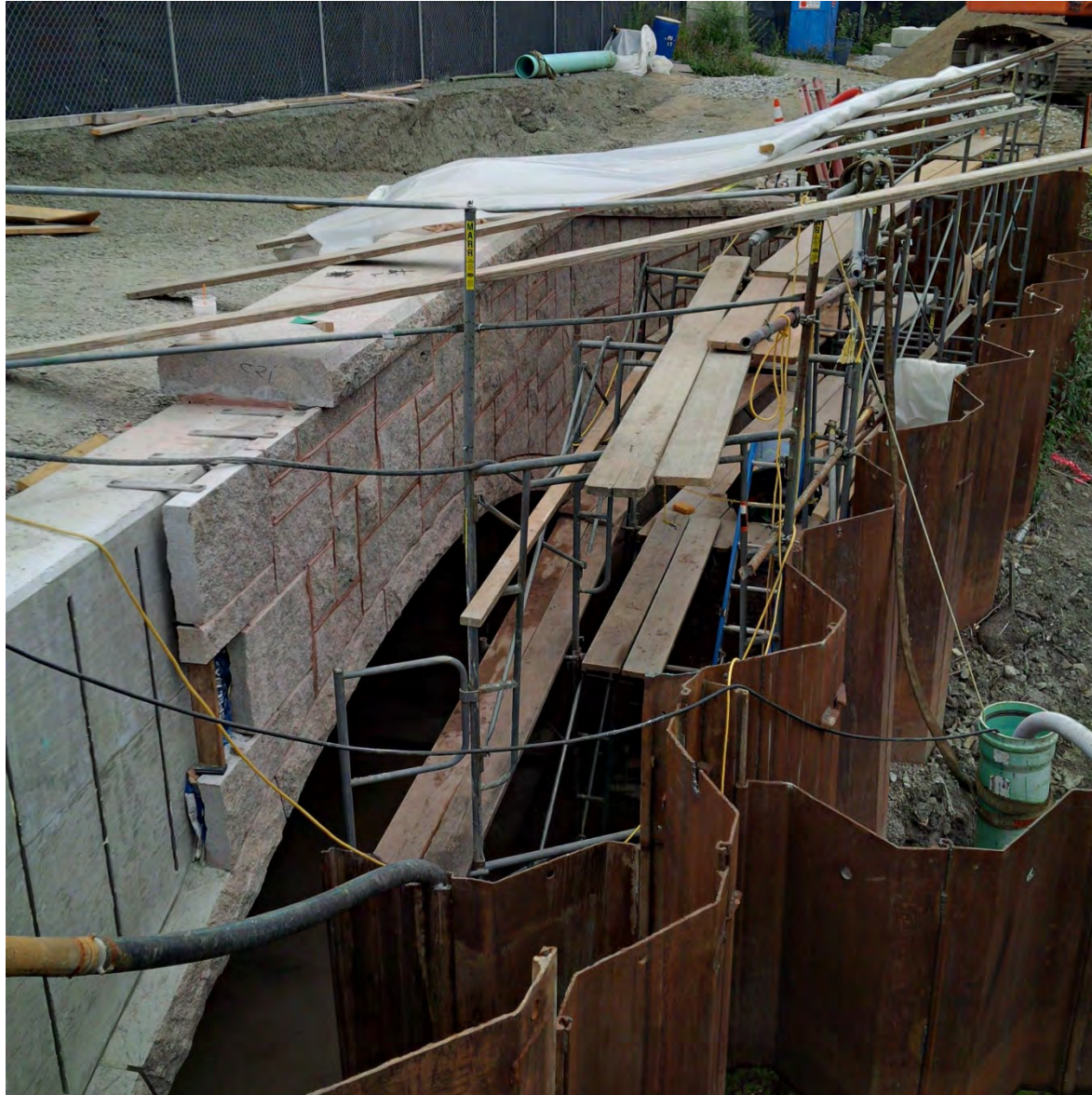
Granite veneer installation and pointing on the upstream headwall of the new Riverway culvert – early September 2015.
